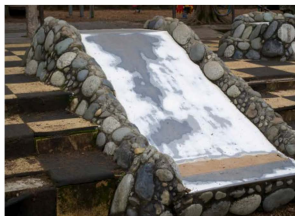
2 Built in Slide/Stonework
