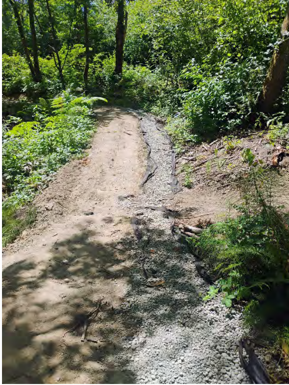
Figure 4 Dispersion trench
