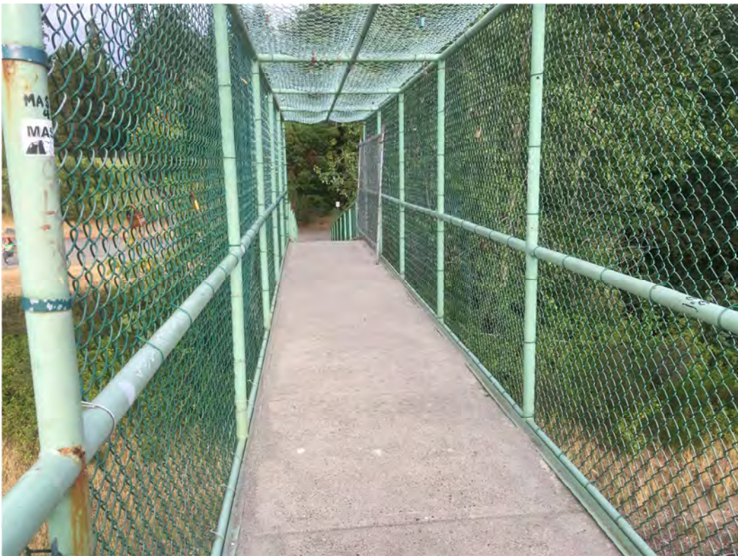
Figure 2 Deck and Fence
