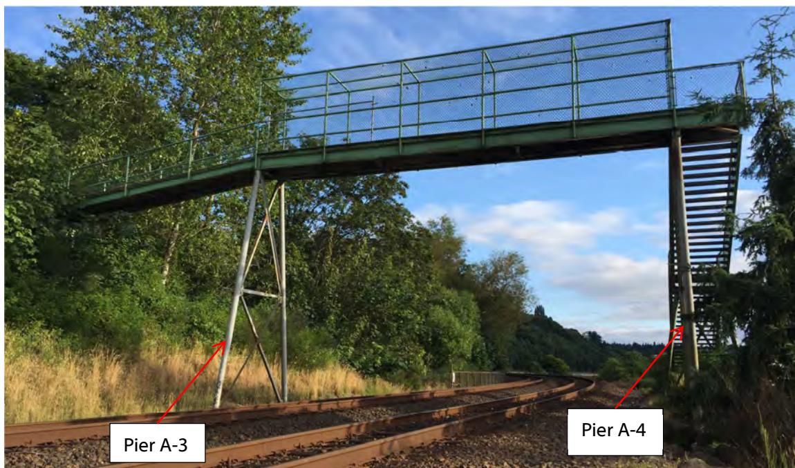
Figure 12 Existing Bridge Pier Locations
