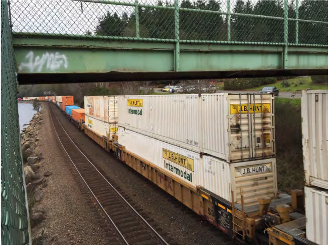
Figure 4 Bridge Low Clearance
