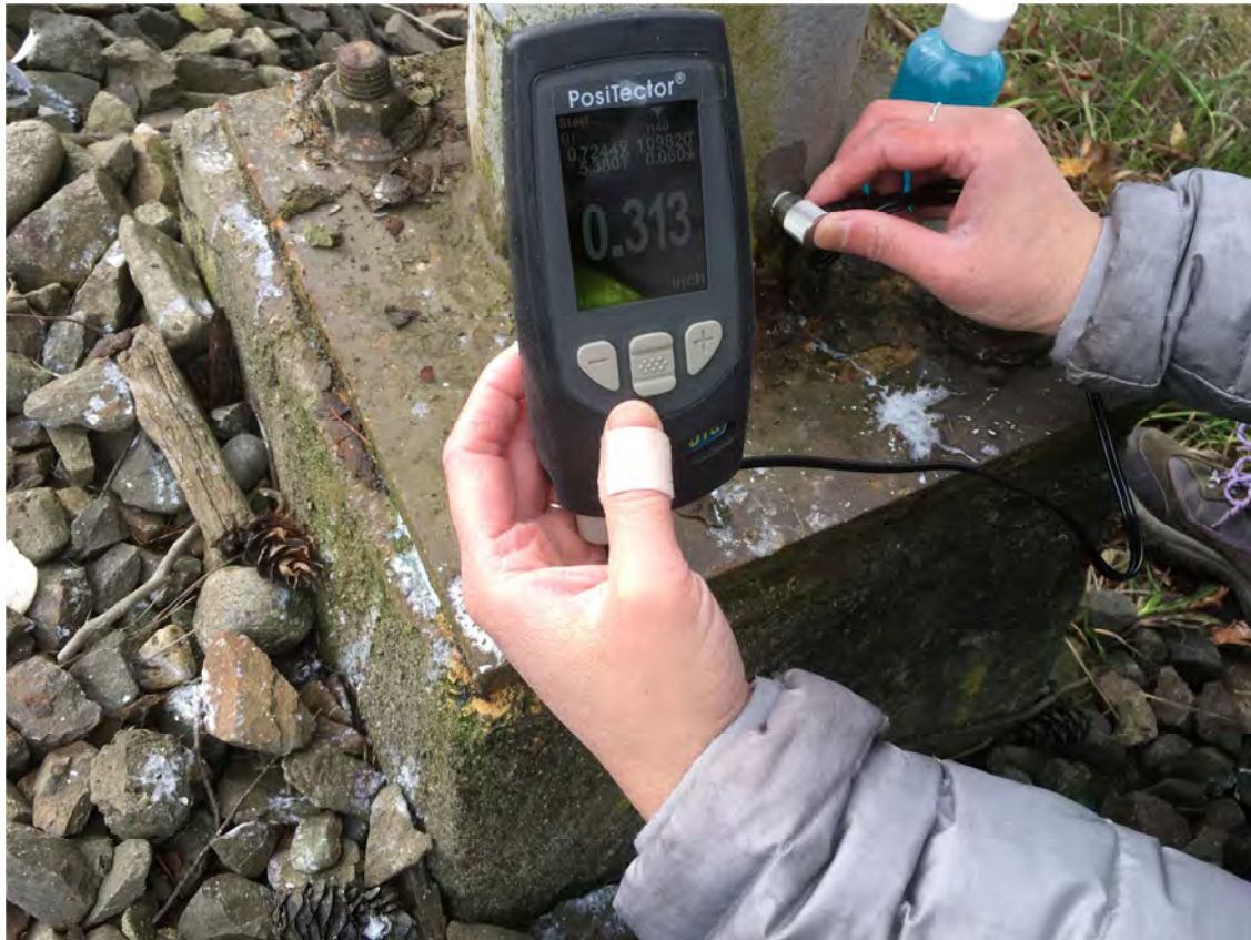
Figure 10 Field Measurement of Steel Thickness
