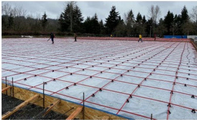
Liner, Formwork, and Reinforcing Cable/Tendons
