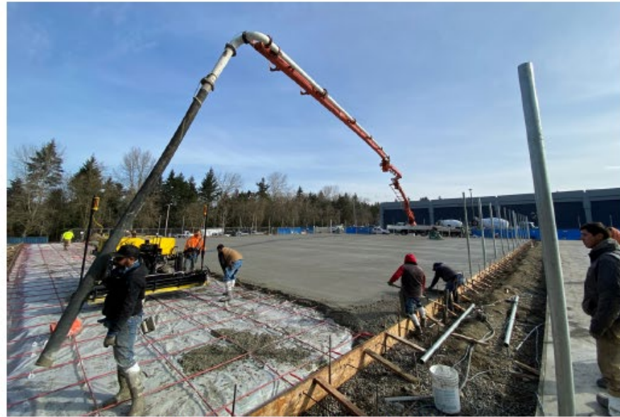
Pump-placement & screeding
