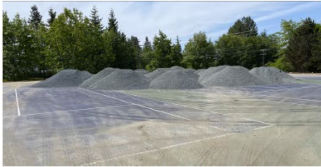
Placing aggregate bedding on failed asphalt tennis courts for a Post-Tension Concrete overlay.
