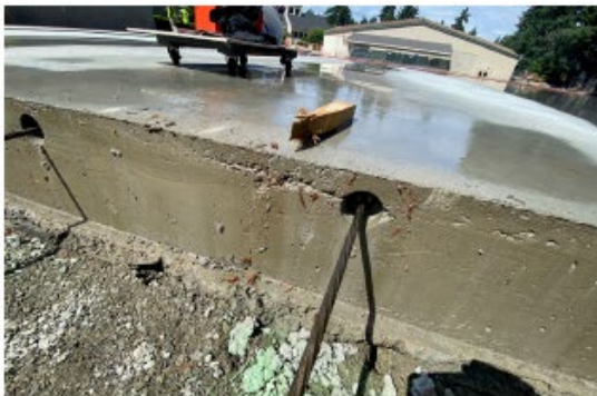
Liner, Formwork, and Reinforcing Cable/Tendons
