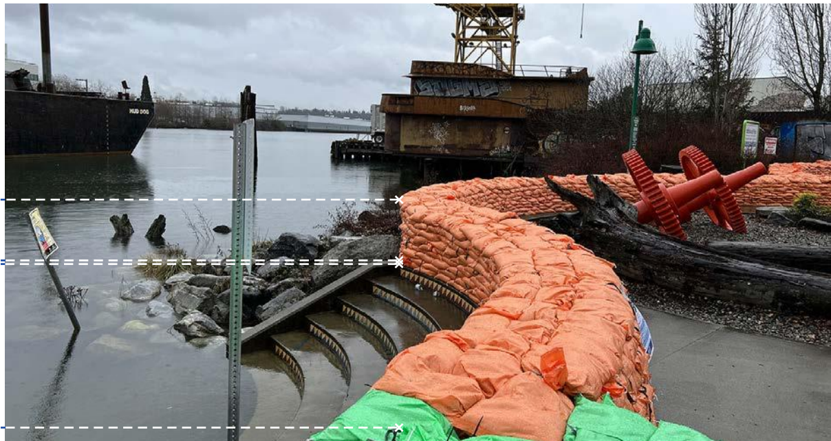
After the December 27th, 2022 flood receded, SPU installed a temporary sandbag berm in low places along the riverbank to protect the community in case of another winter king tide and storm surge. The approximate height of this berm (15 feet NAVD88) is the elevation of expected king tide and storm surge flooding in 2100 with sea level rise. Therefore, protection from flooding in 2100 would need to be about a foot higher than this to ensure full protection.
