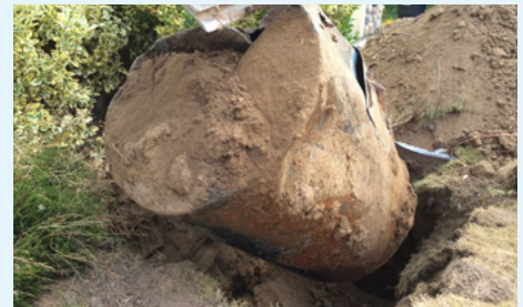
Oil tank being removed from the ground. Photo credit Filco
