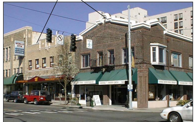
interesting parapets and cornices
