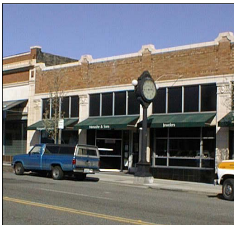
A variety of architectural details including street-level display windows, a sign band, recessed entry, transoms, and facade kick-plates lend human scale and interest to these commercial buildings.
