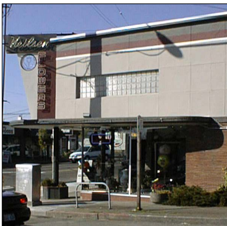
Example of overhead weather protection that is coherently integrated into the building's modern style.
