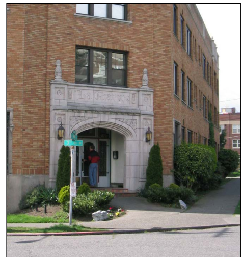
Classical detailing around entrances is a common feature found in the neighborhood.
