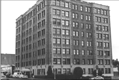
Historical example of midrise building characteristics in the University Community.
