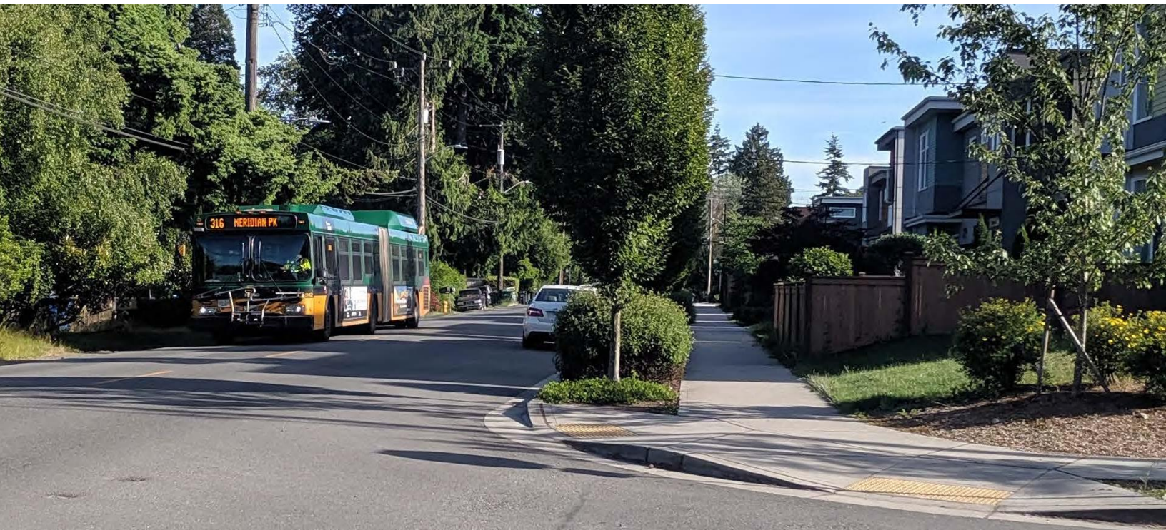
Sidewalk with landscaped buffer along Meridian Ave N at N 140th Street. Source: City of Seattle 130th and 145th Station Area Planning Multimodal Mobility Study, December 2020.
