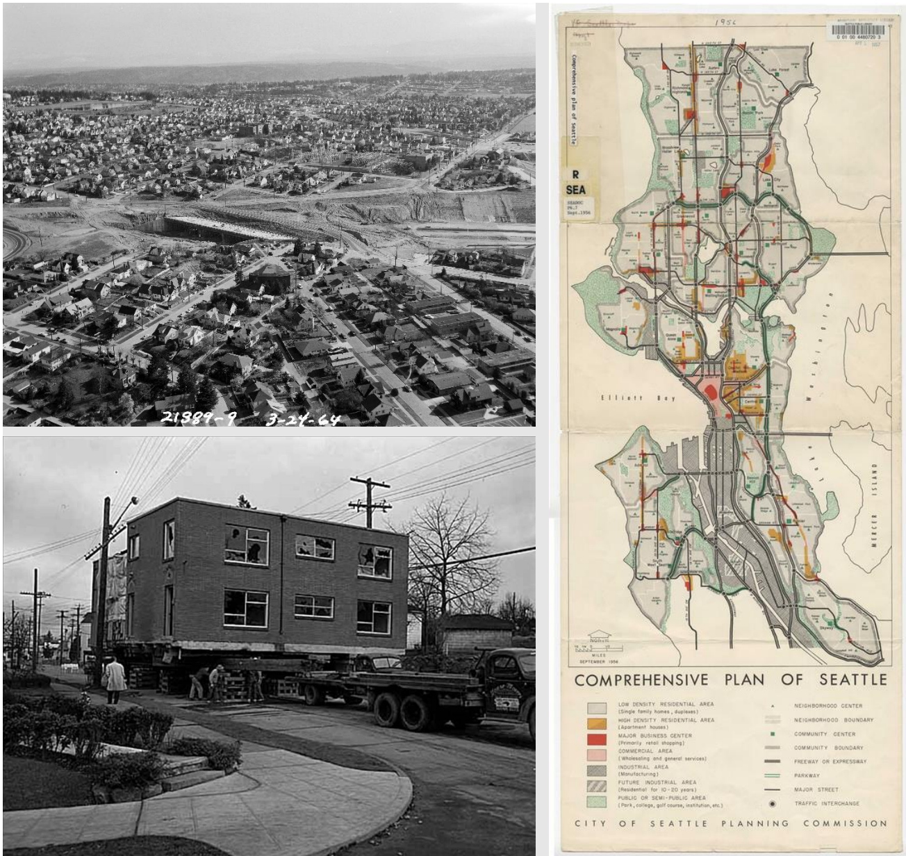
Top left: Construction of I-5, 1964; Courtesy of the Seattle Municipal Archives . Bottom left: Apartment building being moved due to I-5 construction, 1960; HistoryLink Essay 4168 via MOHAI (1986.5.4007). Right: City of Seattle 1957 Comprehensive Plan; Seattle Public Libraries Special Collection.
