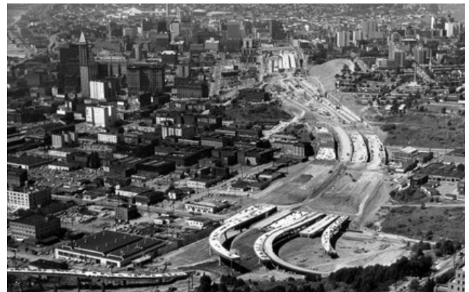
The construction of I-5, looking north from Beacon Hill. (WSDOT Photograph Collection: Washington State Archives)
