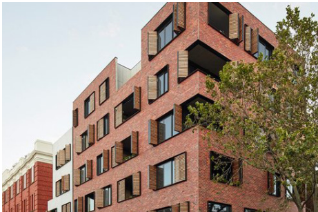
The use of bricks evoke a sense of durability, permanence, and fine-grained complexity. Punched windows with operable shutters add depth and scale with an ever-changing facade.
