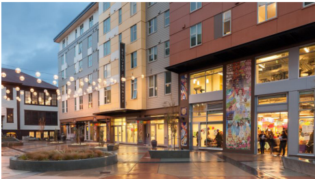
A courtyard plaza connected to the sidewalk provides a space for seating, food kiosks, community and cultural events and festivals.
