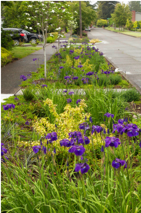
A wide planting strip with Green Stormwater infrastructure provides habitat, reduces runoff, and contributes to a visually-engaging and comfortable walking experience.
