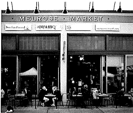
Restaurant storefront that engages with the public sidewalk and street.
