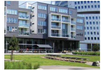
Building mass and modulation can open up a plaza or open space to sun and air. Image courtesy of Schemata Workshop.
