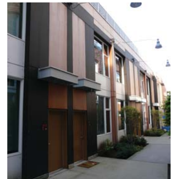
A modern example of ground-related housing. Alley 24 Seattle.
