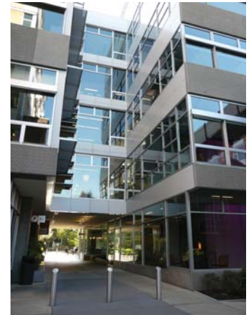
An example of a midblock crossing that retains buildable space above. Alley 24 Seattle
