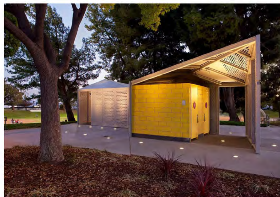
Clover Park - Santa Monica, CA Shared lavs Natural ventilation + daylight Privacy screening/ Views out Full height stall walls w/minimal space below door Bright colors
