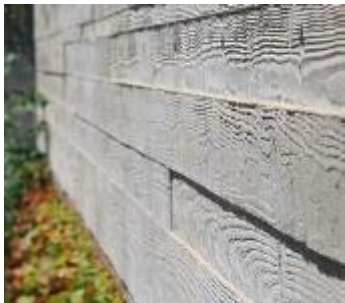
adze texture concrete walls
