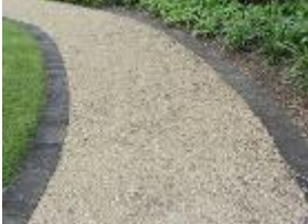
gravel pathway with concrete edging
