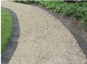
gravel pathway with concrete edging
