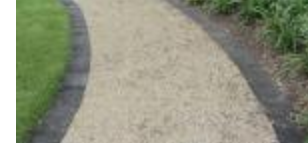
gravel pathway with concrete edging
