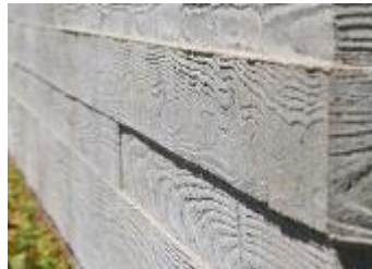
adze texture concrete site walls
