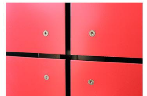
Type 3A - Pre-Finished Aluminum Plate Cladding with Exposed Fasteners
