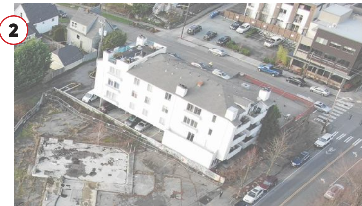
2 Mixed Use Residential Building
