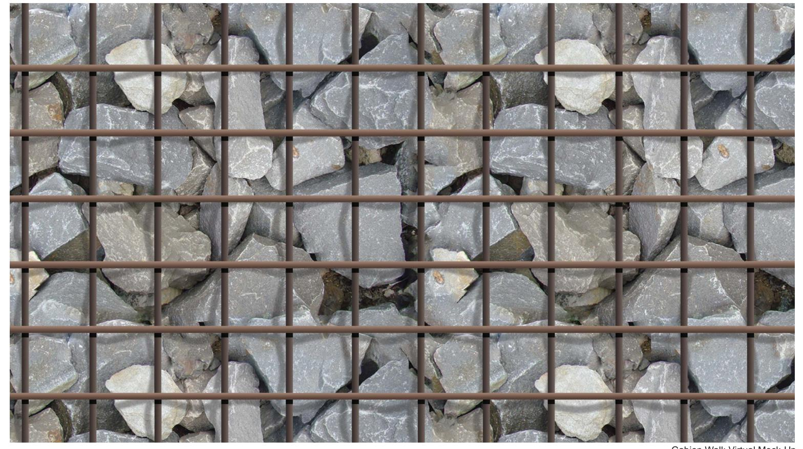
Gabion Wall: Virtual Mock-Up 4"-8" Basalt Fill with 3/8" Welded Wire at 4" Spacing On Center
