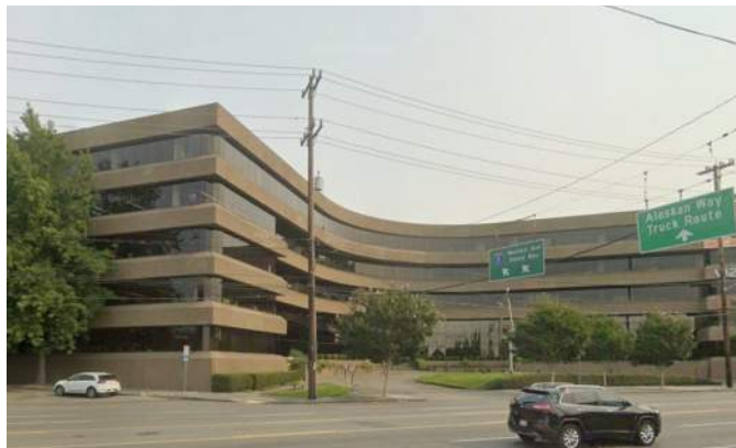
(E) * 300 Elliott Ave W (Office)
