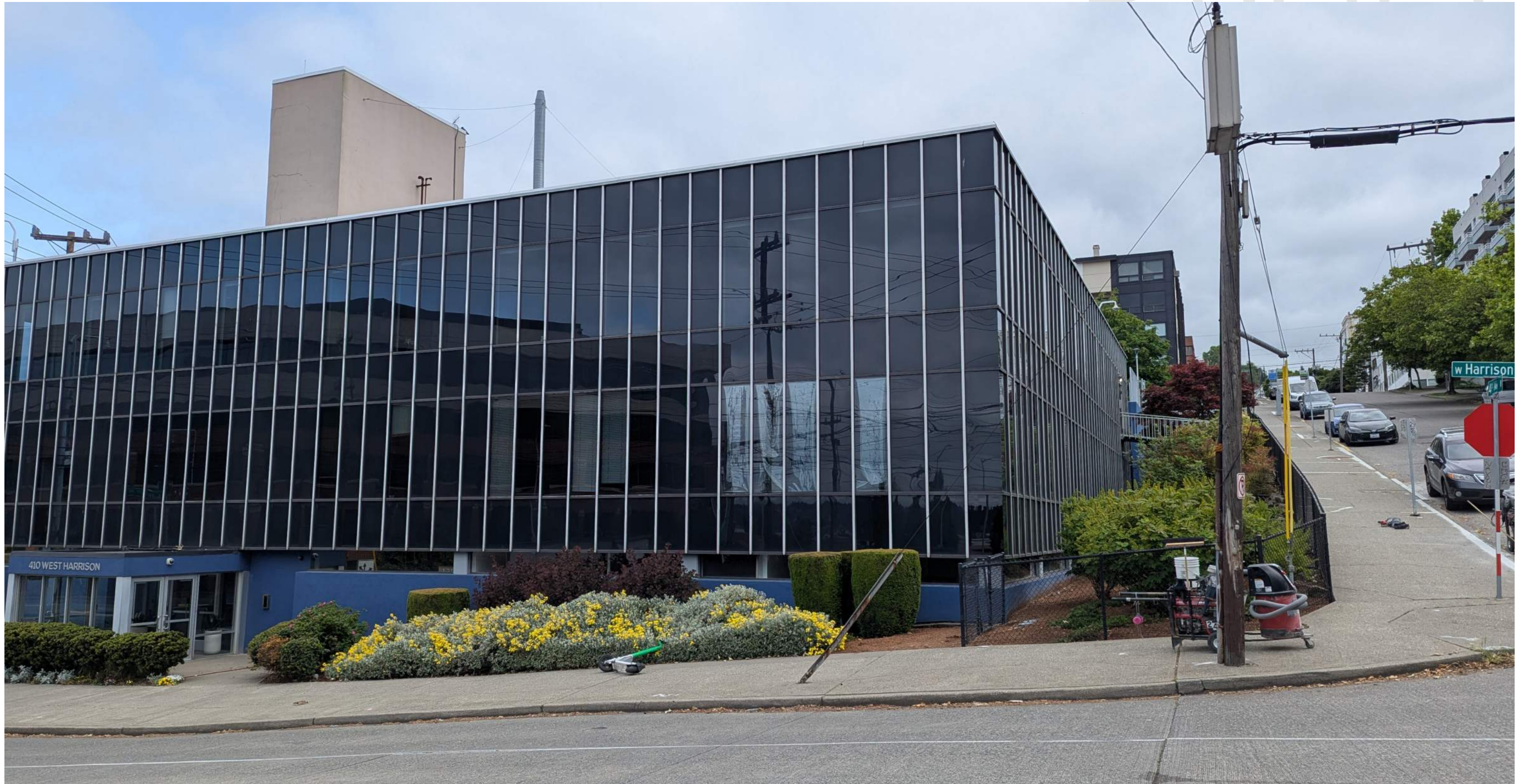
VIEW LOOKING NORTH AT HARRISON ST & 4TH AVE
