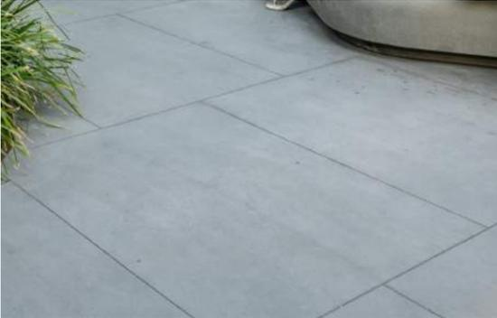
Concrete Paving, Integral Color, Saw-cut Joints, Sandblast Finish
