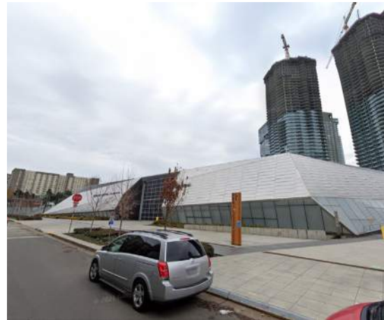
⑦ Denny Substation
