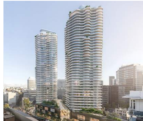
⑧ 1200 Stewart Street (Under Construction)
