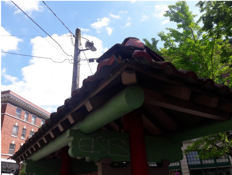
Kiosk: Replace roof; other repairs as needed $10,000
