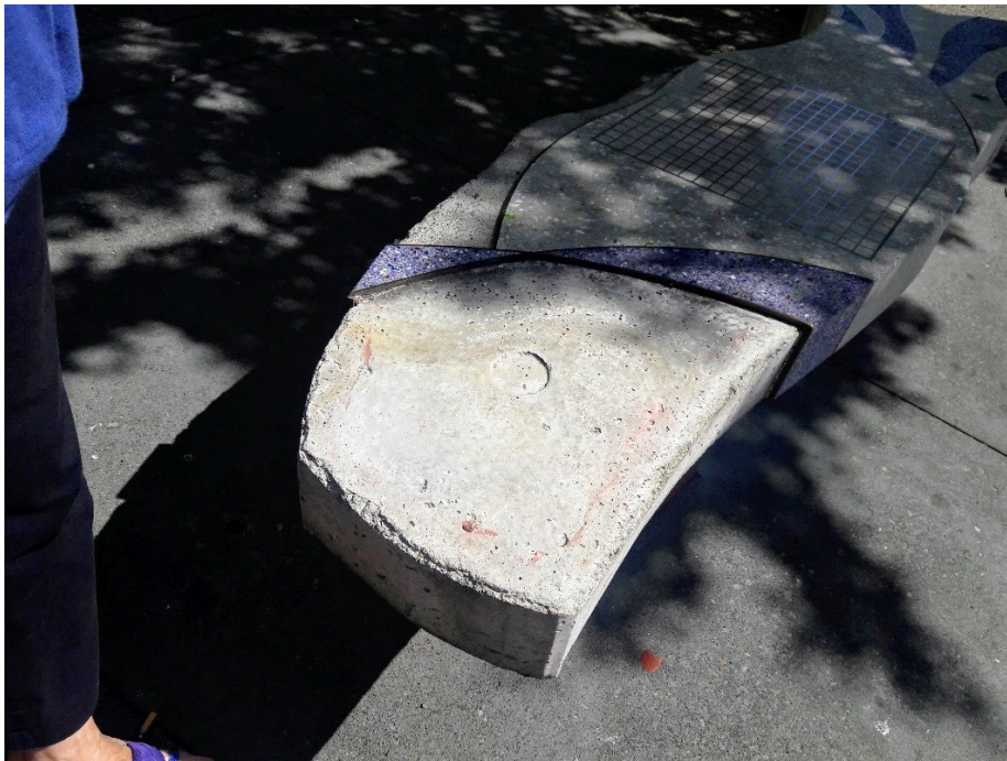
Art benches along S King ST: repair terrazzo tiles (new handrails will protect benches from skaters)- $6,000
