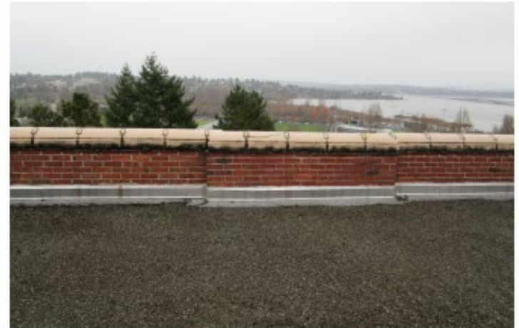
PHOTO OF PARAPET
