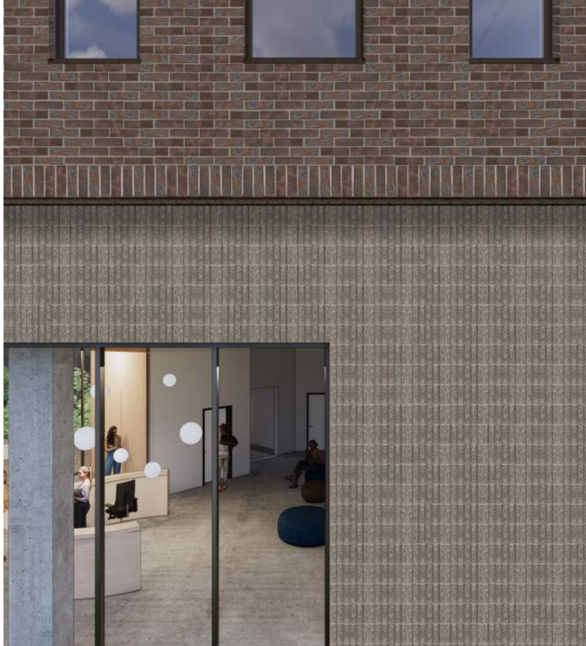
BRICK UPPER VOLUME AND SCORED CMU BASE
