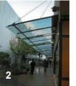
2 • Glass awning - allows light to pass thru; but dirt visible from below
