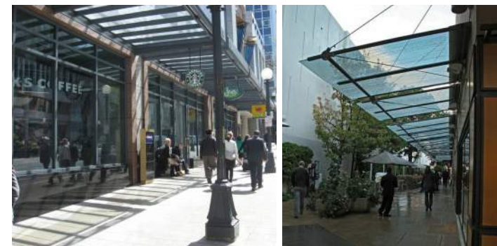
Transparent/Translucent sidewalk canopies offer protection from rain while allowing sunlight to shine through.
