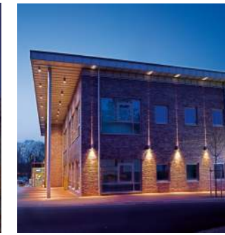
Building-mounted lighting brightens the sidewalk
