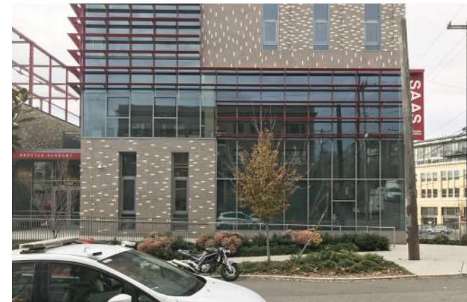
Gray and white brick create a visual texture, glass with red sun shades span the facade to break-up the massing
