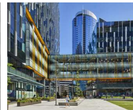
Transparent skybridge offers visual connections in and out of building
