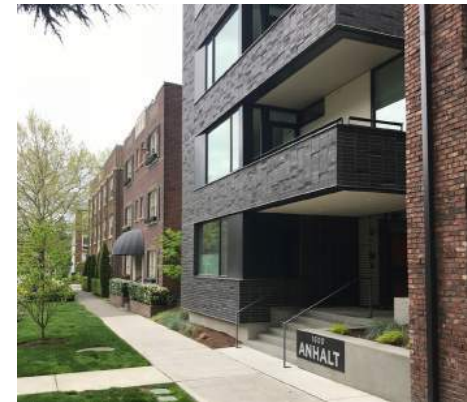
New construction references adjacent building through choice of materials, rhythm, and scale
