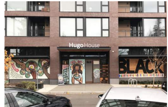
Red-brown brick with black framed storefront windows and wood accents above ground level - wood accents reduce the visual weight of the brick
