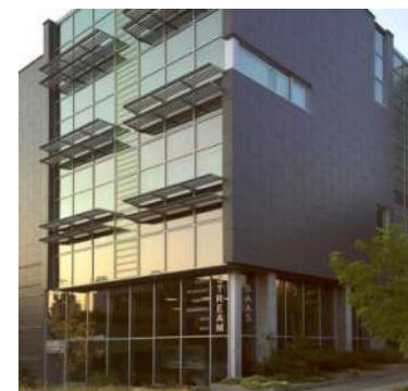
Physical expression of sustainability measures. Sun shades reduce solar gain and reduce cooling needs
