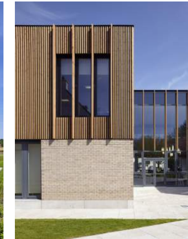
Transparent building entry framed by brick massing
