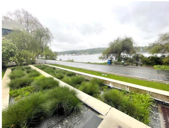
Regional Stormwater Facility at UW Harris Hydraulics
