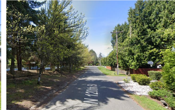
N 120 th St Existing View – Northeast Edge
