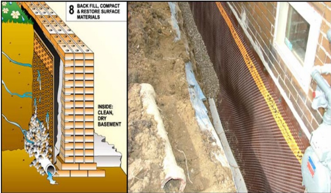
IMAGE 04: PROPOSED DRAINAGE AT EXISTING BRICK FOUNDATION
