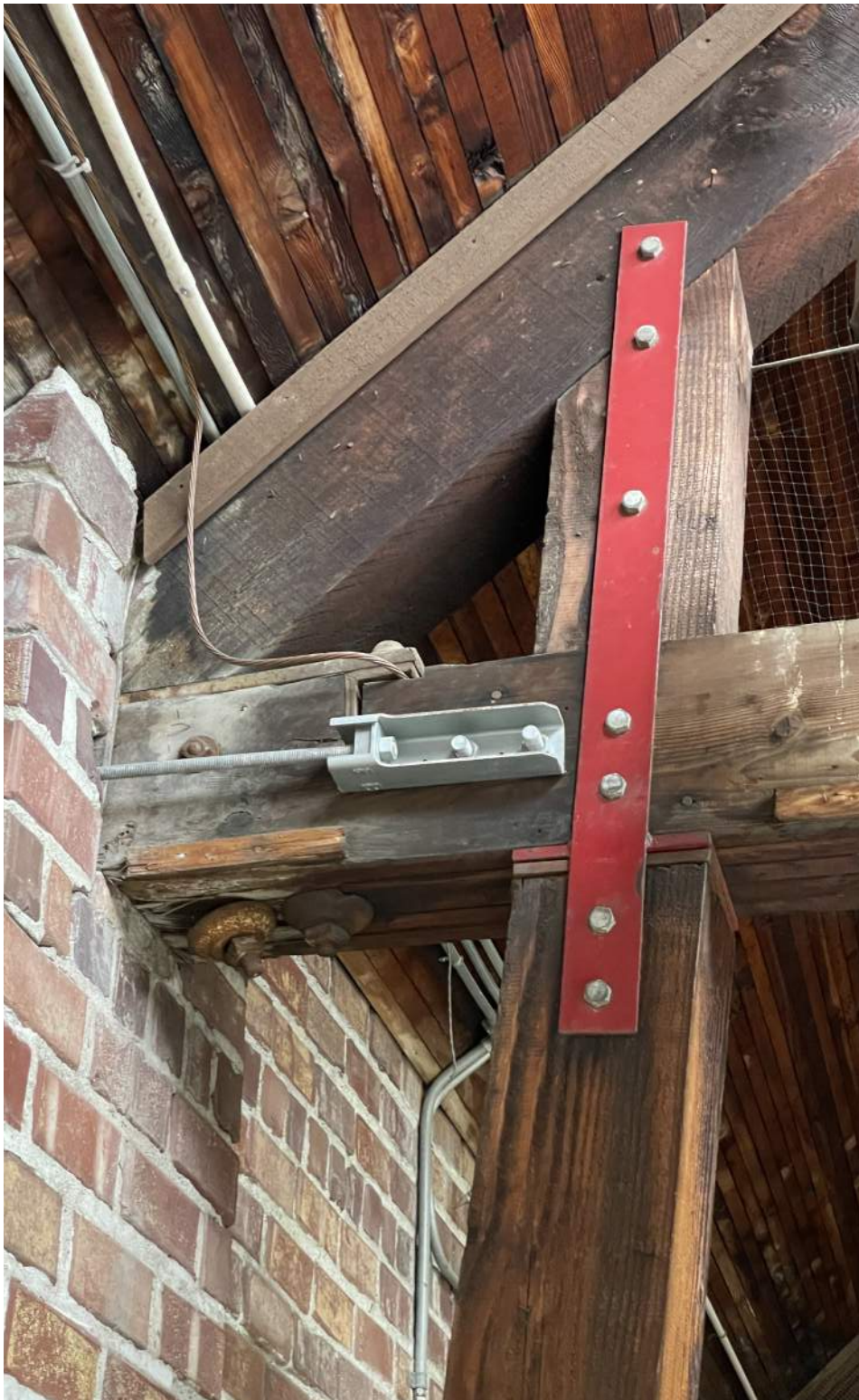
EXISTING TRUSS TIMBER SUPPORT AT PILASTER
