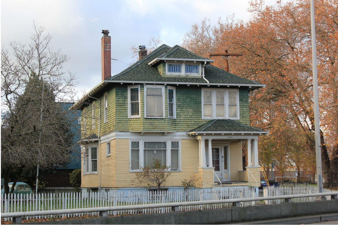
B1. Woodin House, view NW from Corson Ave S exit ramp
