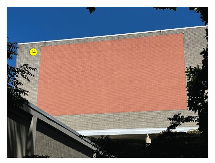
**Condition 14:** Vinyl banners attached to existing wall brackets and wiring on south façade of fly loft
