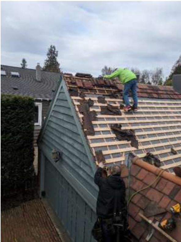
Garage Roof (repair work & finished product):
