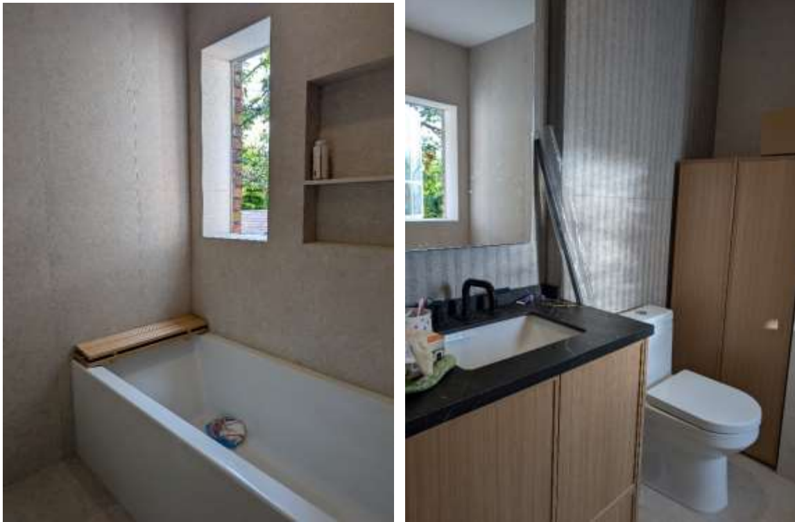
2 nd Floor new bathroom #1 (finished product):
