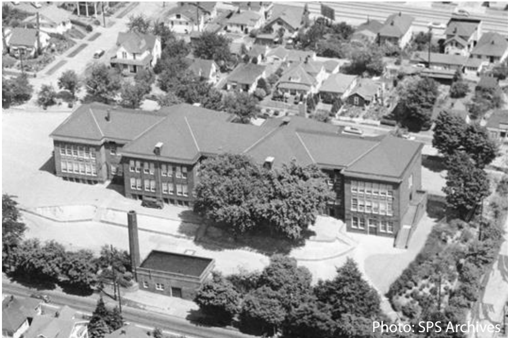
AERIAL VIEW FROM WEST SHOWING 1916 ADDITIONS
