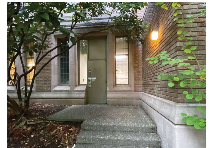
Southeast entry added in 1971.
