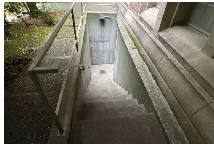
Tunnel access stair added in 1971
