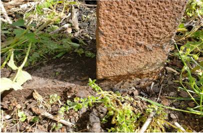
2. The southwest vertical support element is badly corroded that the steel material is peeling off, therefore reducing the effective strength of this element.
