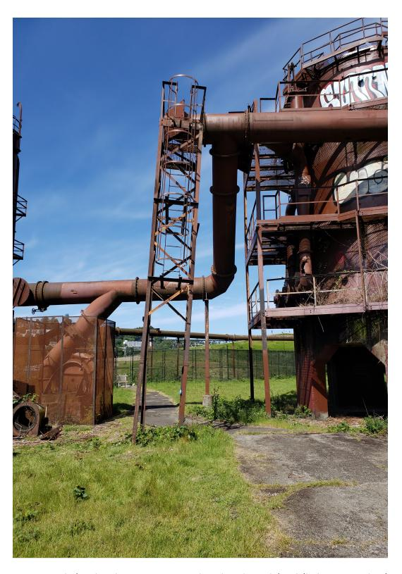
It is my recommendation that the tower structure be taken down. It is a failed structure that is unsafe to be left at its current condition/position. It is not recommended to be rebuilt or refurbished because its elements are deteriorated and badly corroded. The demolition of this tower must be done as soon as possible.
