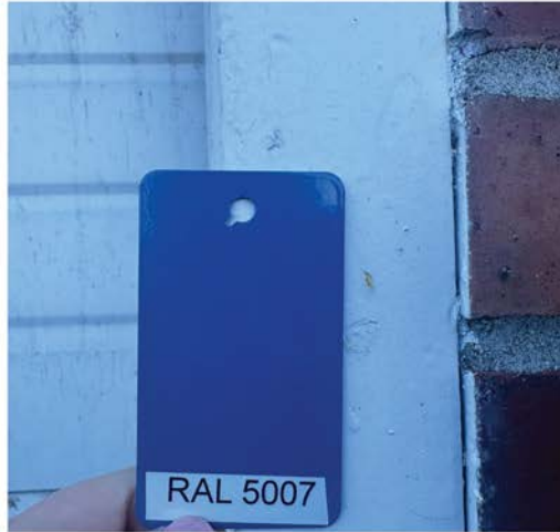
at location of proposed door replacement
