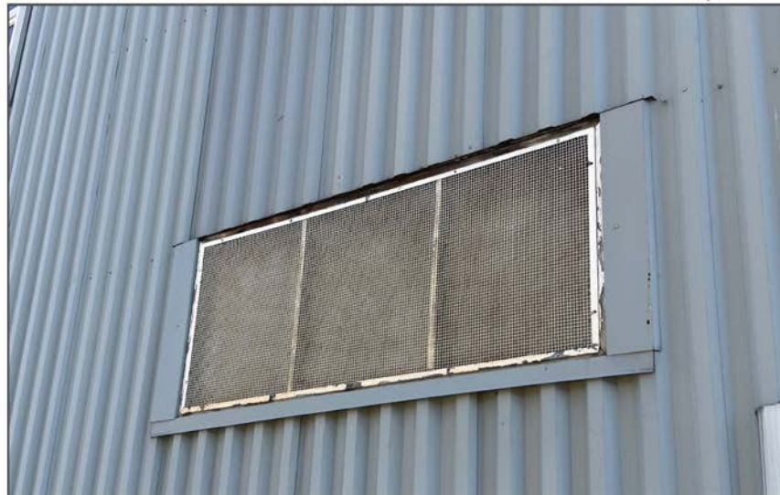
Figure 20 • Detail of screen vent to be re-used
