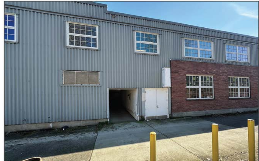
Figure 18 • Western facade opposite loading dock, area of proposed new HVAC installation
