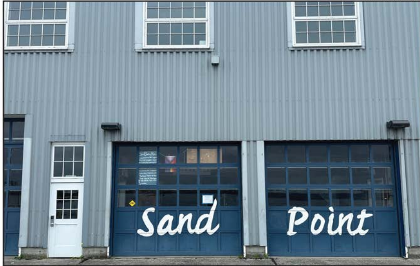
Figure 11 • Eastern facade, detail of Sail Sandpoint roll-up doors
