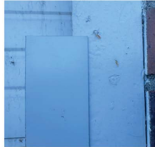
at location of proposed door replacement
