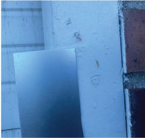
at location of proposed door replacement
