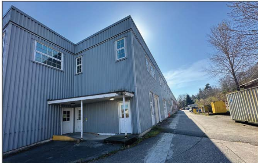
Figure 16 • western end of northern facade viewing south down western facade at alley
