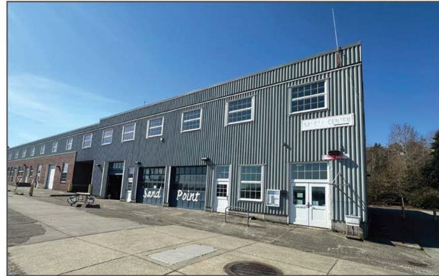
Figure 13 • Northern end of eastern Facade
