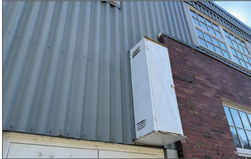
Figure 19 • Detail of unit to remain
