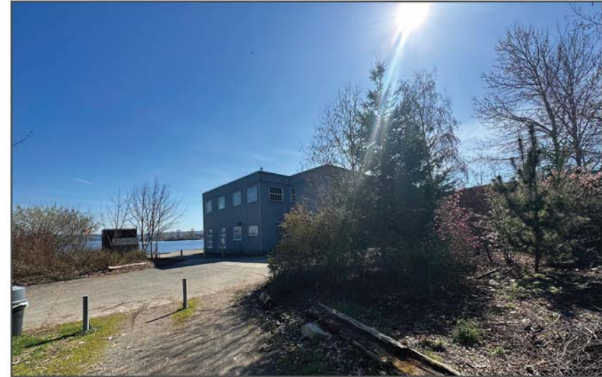
Figure 21 • View of western facade from approach at trail
