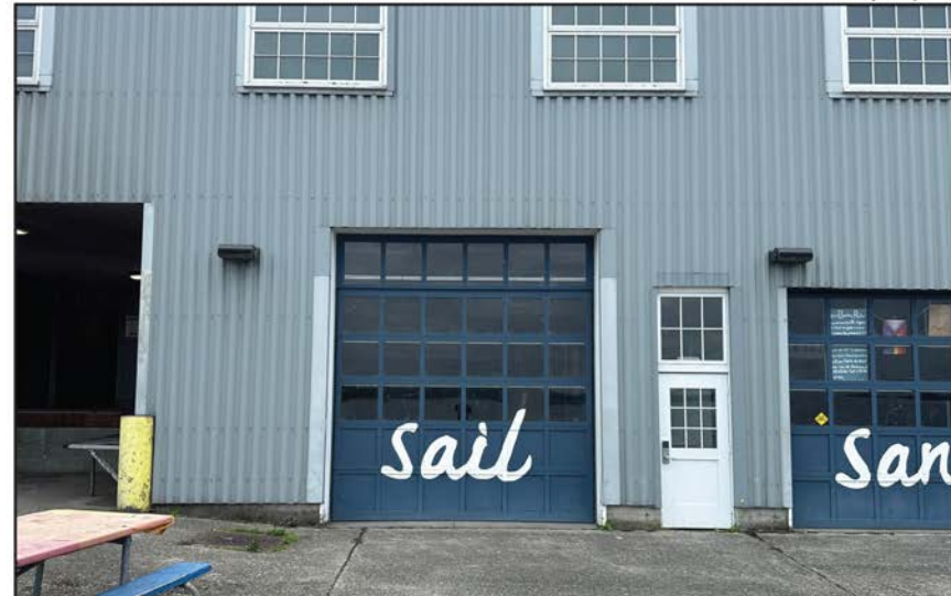
Figure 10 • Eastern facade, detail of Sail Sandpoint doors, southernmost roll-up door and mandoor
