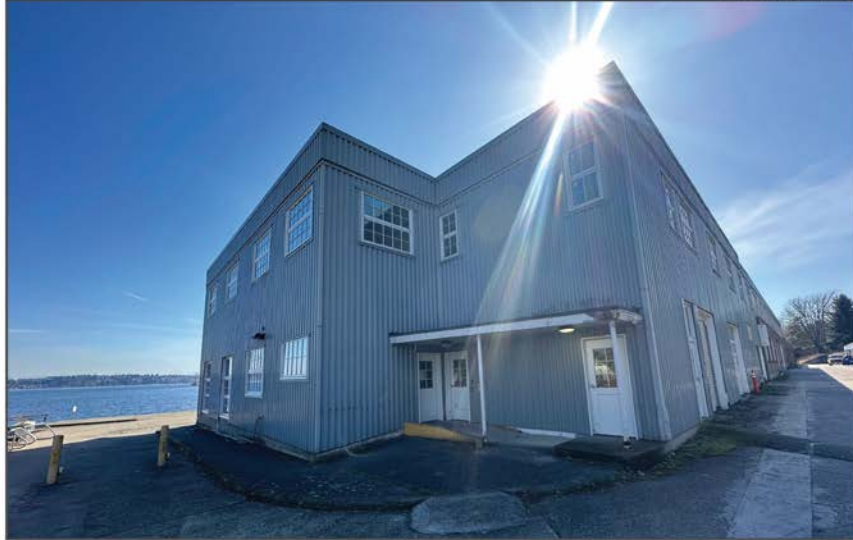
Figure 15 • Northern facade viewing southeast
