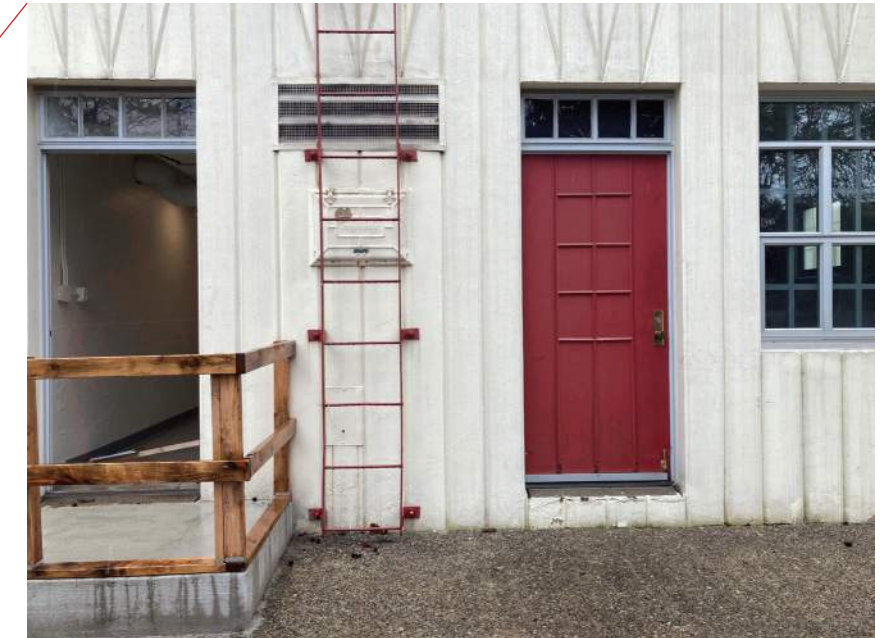
figure 38: Existing steel components painted red
