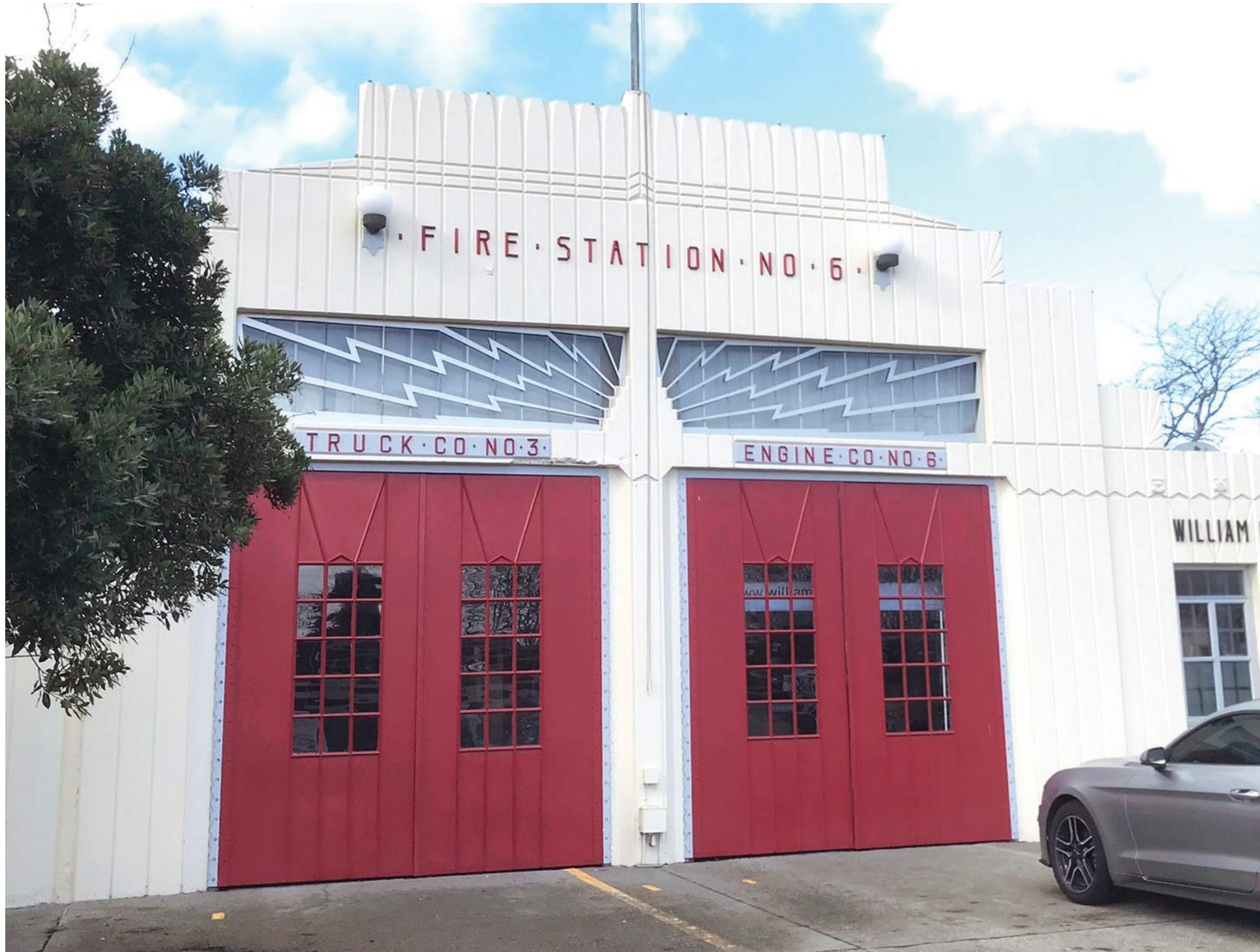
figure 35: Current condition of apparatus bay doors, 1986 replica of original
