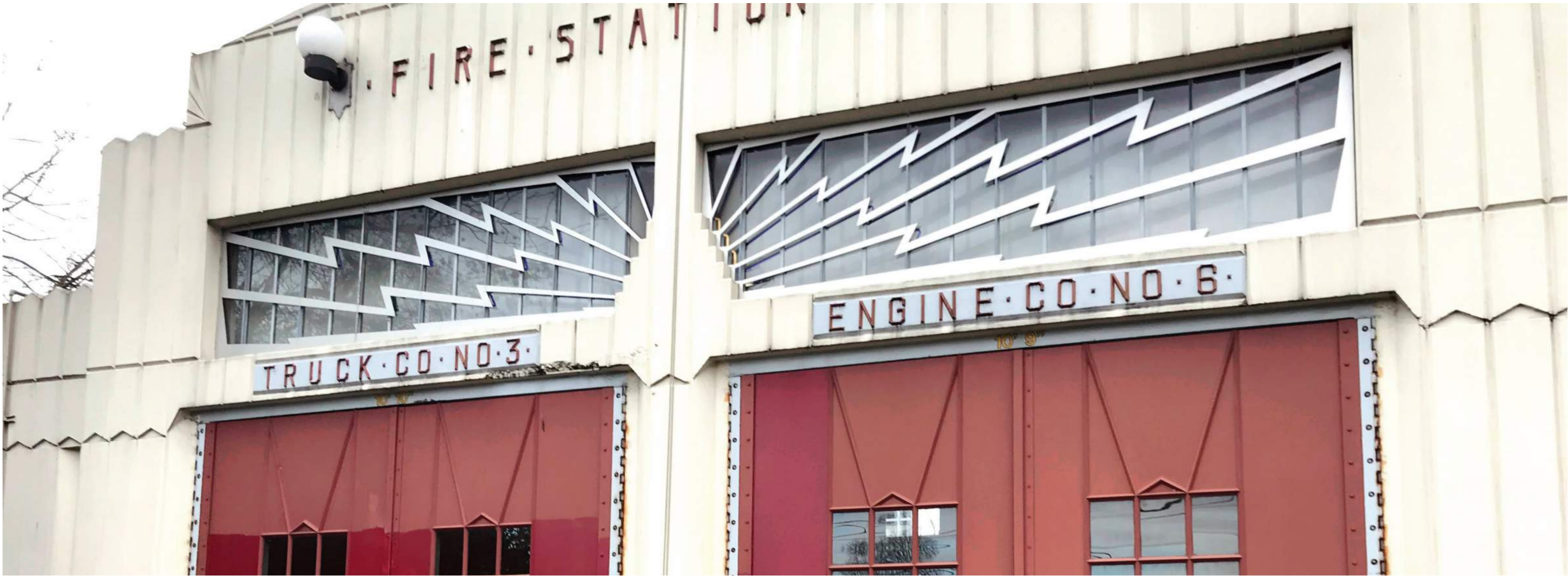
figure 36: Original 1931 steel sash windows with 1986 replica "lightning bolt" grill
