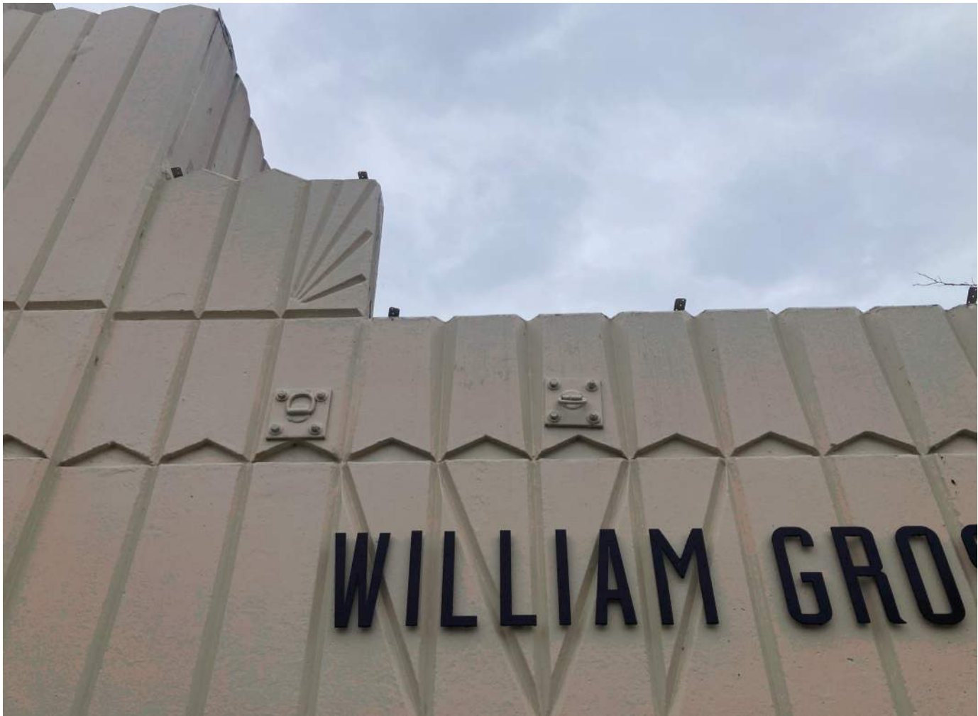
figure 5: Image of Art Deco profile at parapet.
