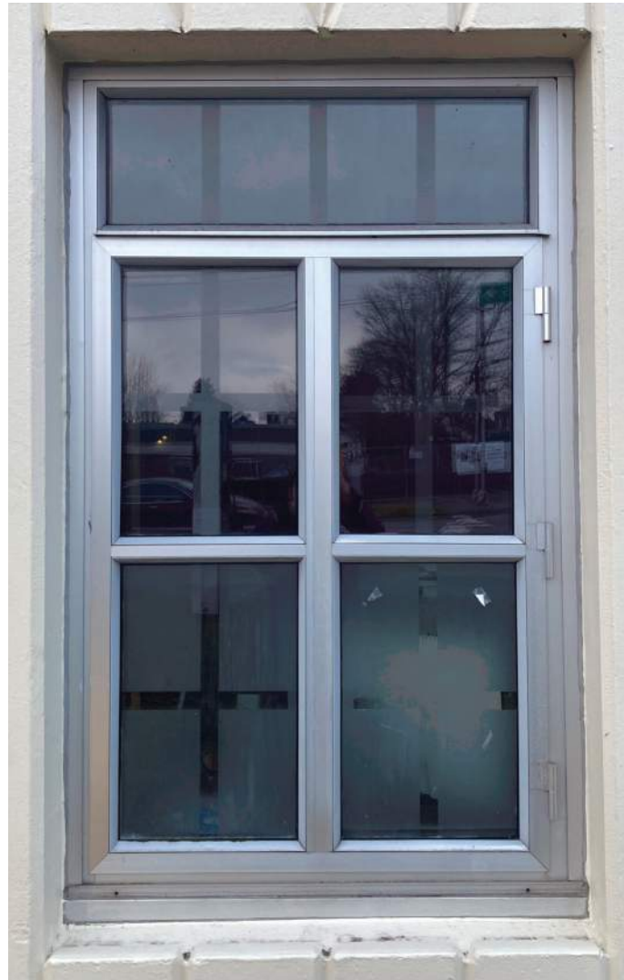
figure 12: Existing 1999 aluminum window with etched "panes."
