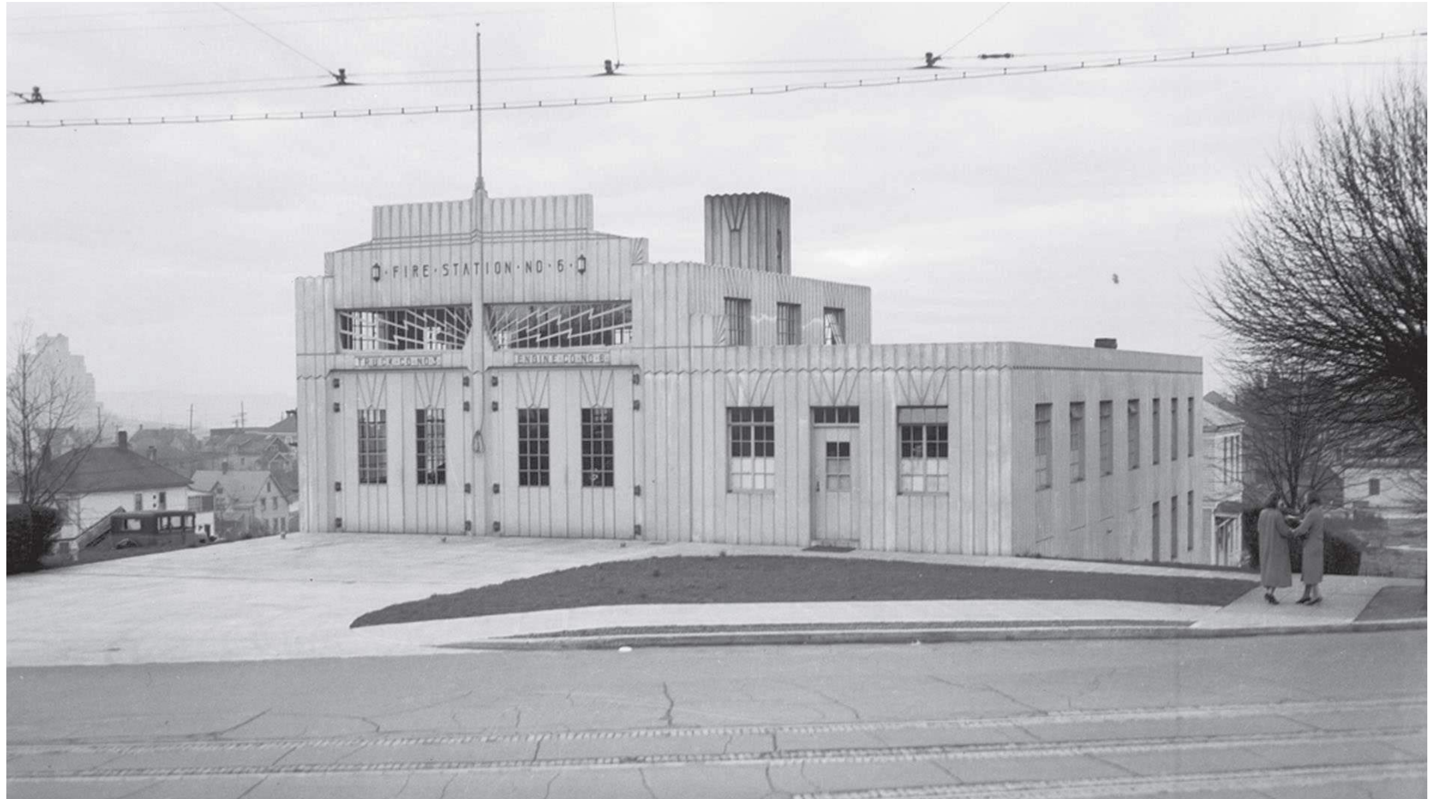
figure 1: Historic photo showing apparatus bay doors, lightning bolt window, and typical windows.
