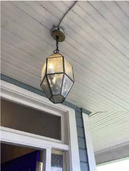
EXISTING LIGHTING FIXTURE
