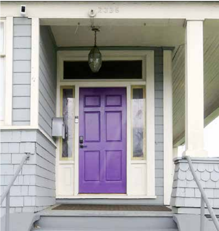
EXISTING LIGHTING FIXTURE AT ENTRY
