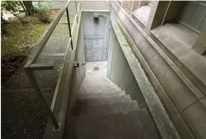
Tunnel access stair added in 1971
