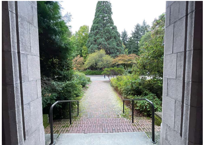
Non-historic painted metal handrail
