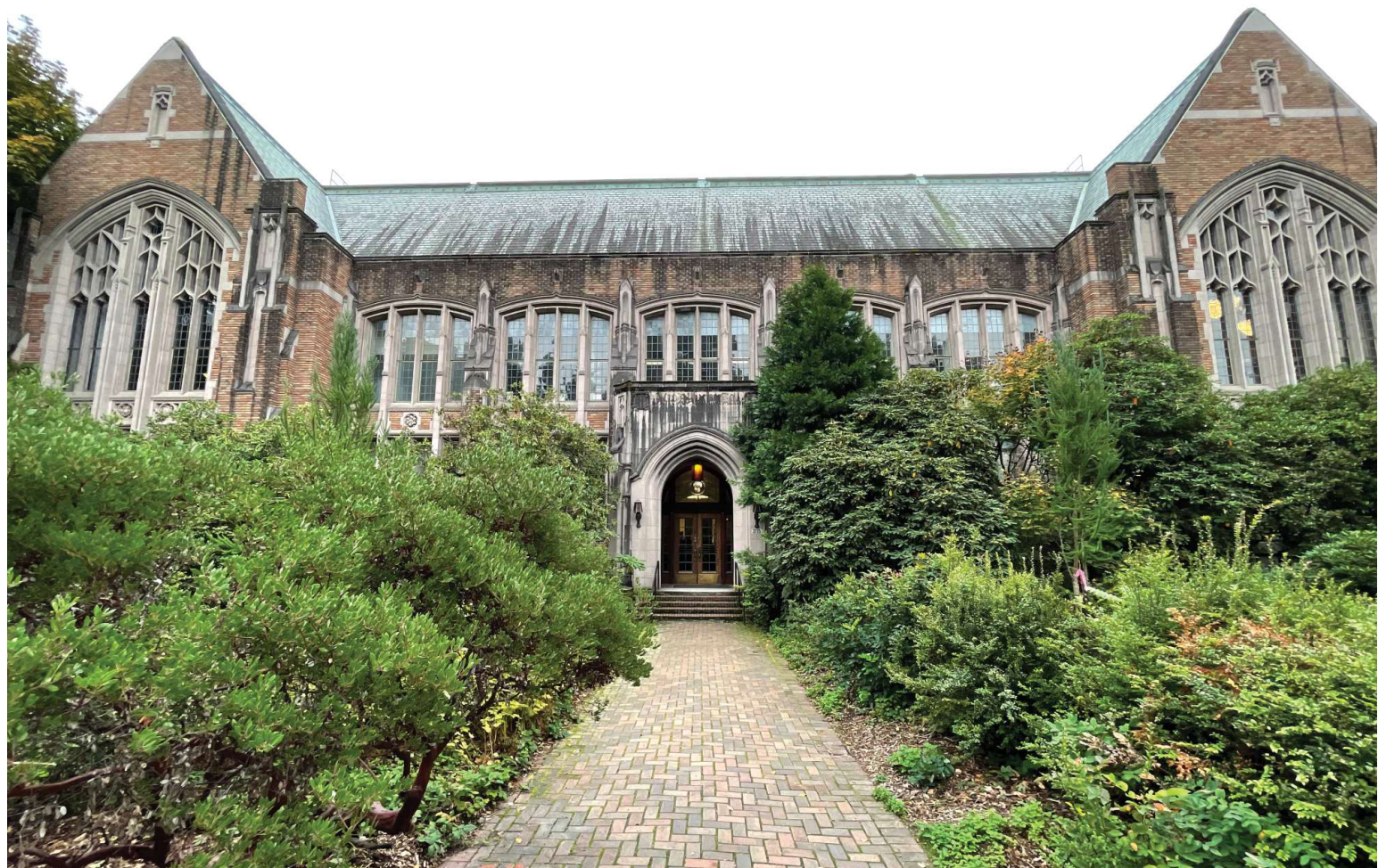
North elevation, entry walkway, and landscaping
