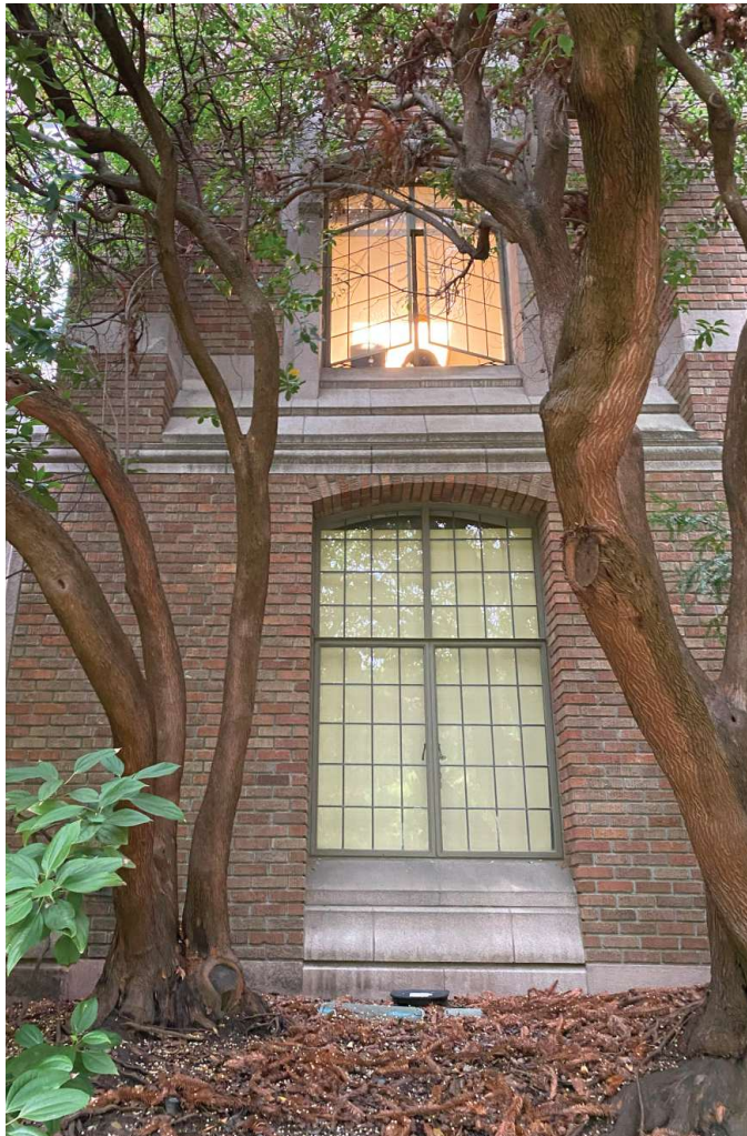
Replacement window at historic south entry
