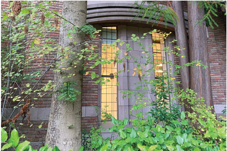
1971 infill at southeast wing
