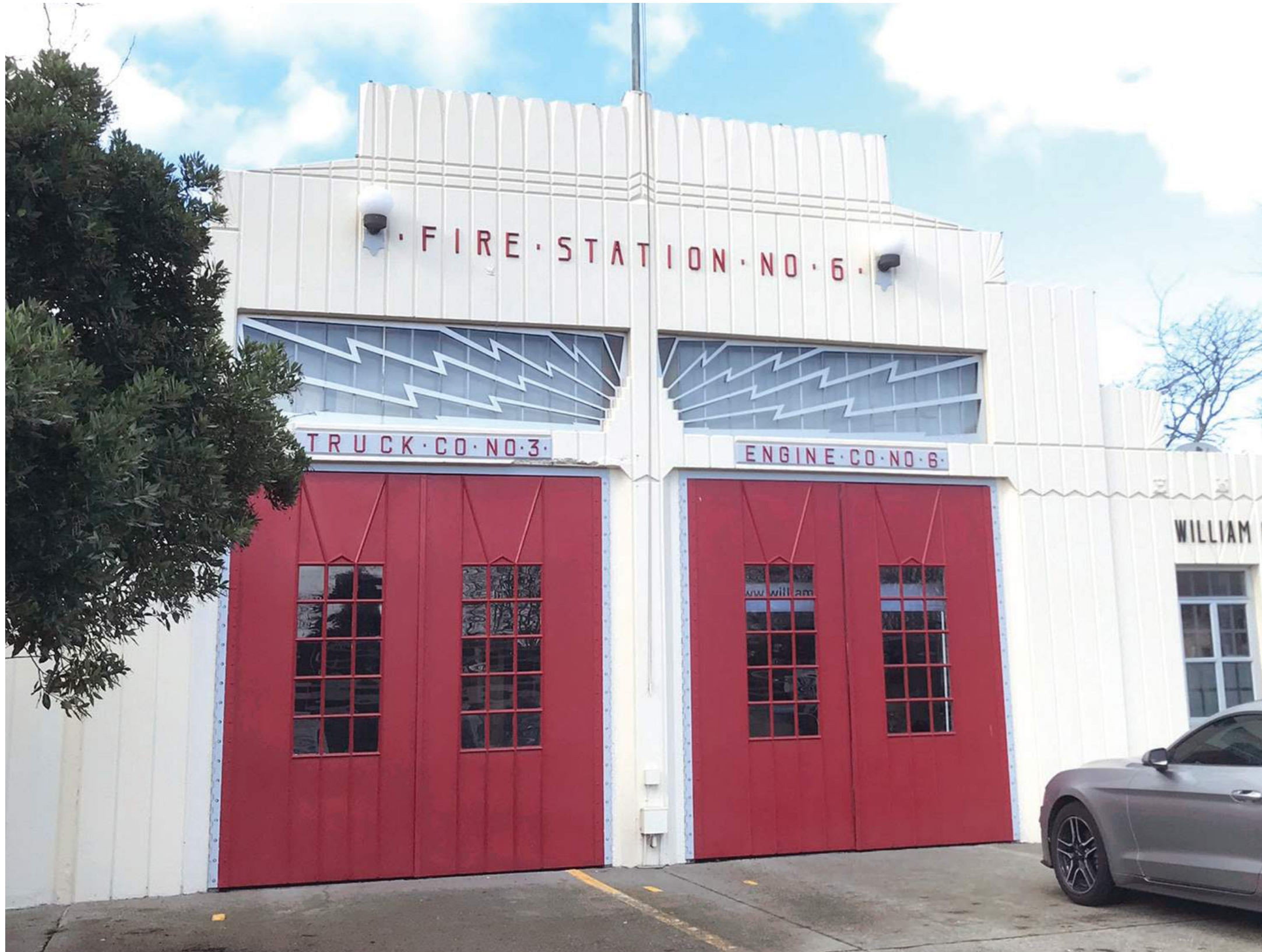
figure 34: Current condition of apparatus bay doors, 1986 replica of original
