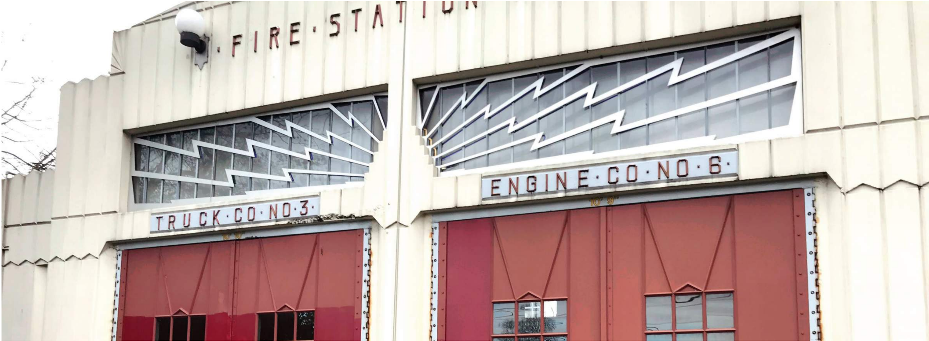
figure 35: Original 1931 steel sash windows with 1986 replica "lightning bolt" grill
