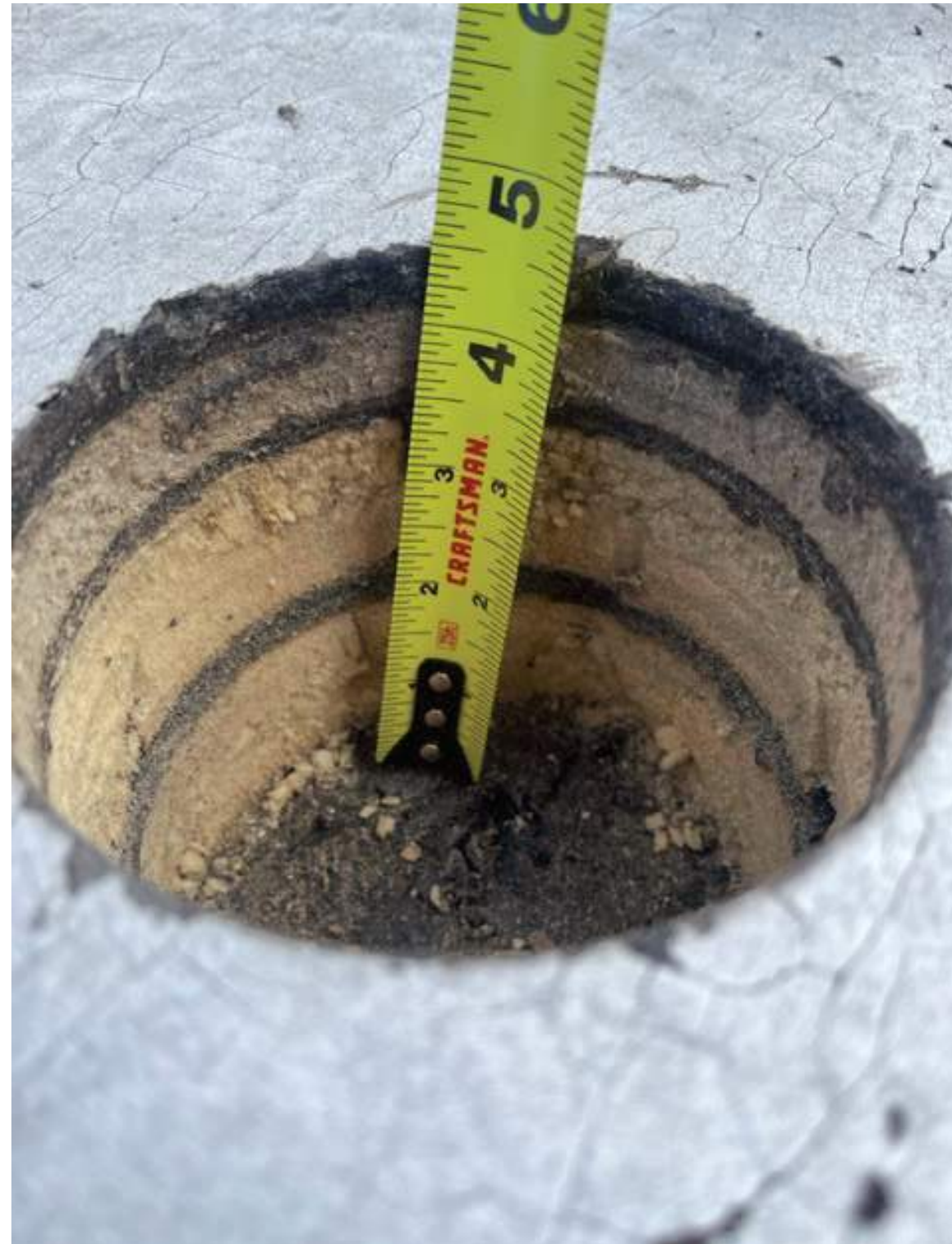
figure 6: Core taken from current roof shows 4.5" of insulation.
