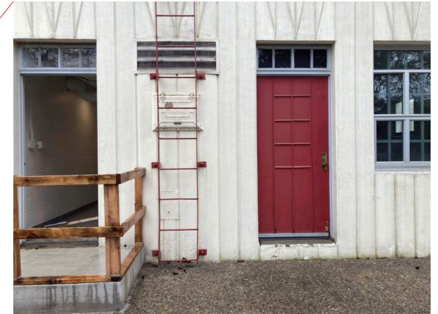
figure 37: Existing steel components painted red
