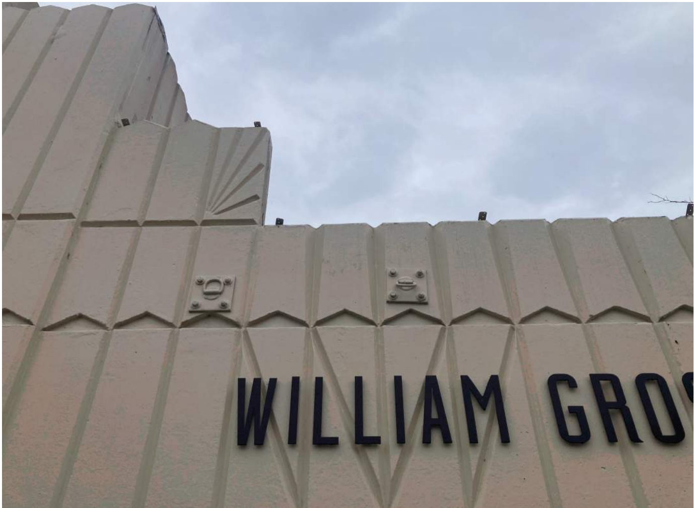
figure 4: Image of Art Deco profile at parapet.
