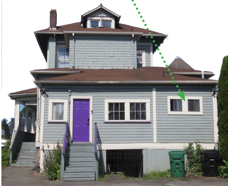
EXISTING RESTROOM WINDOWS (#103 & #104)
