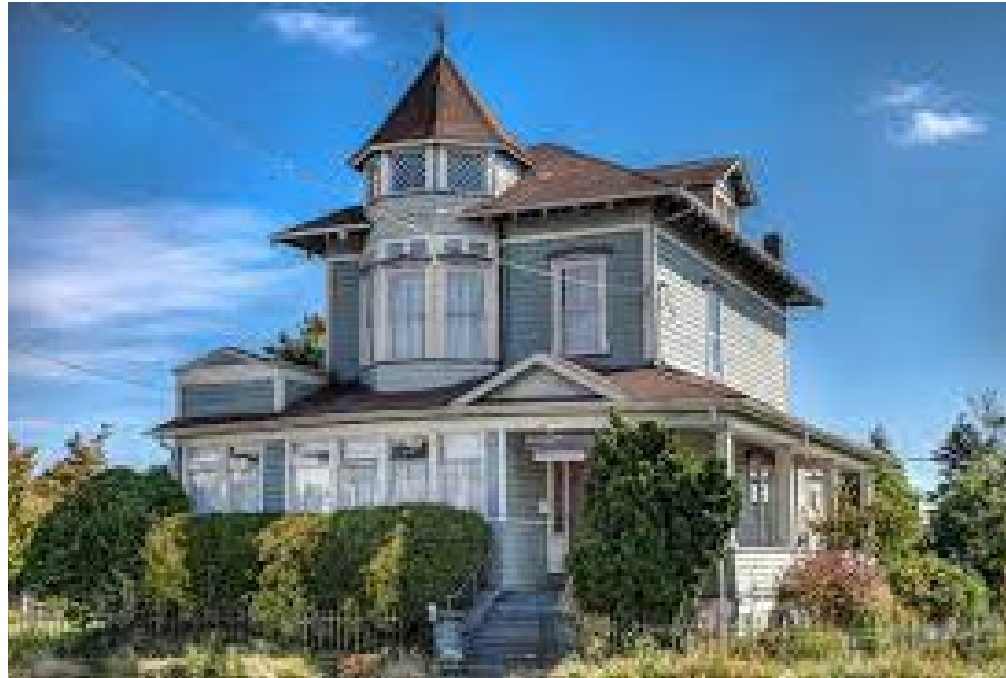
EXISTING BUILDING EXTERIOR
