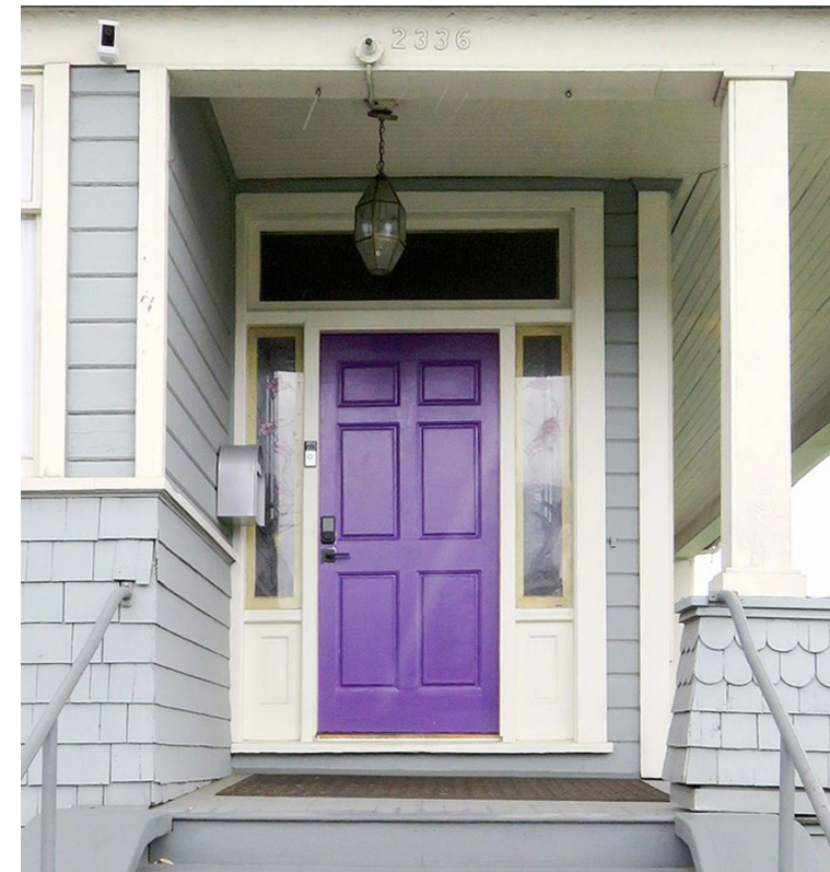
EXISTING LIGHTING FIXTURE AT ENTRY
