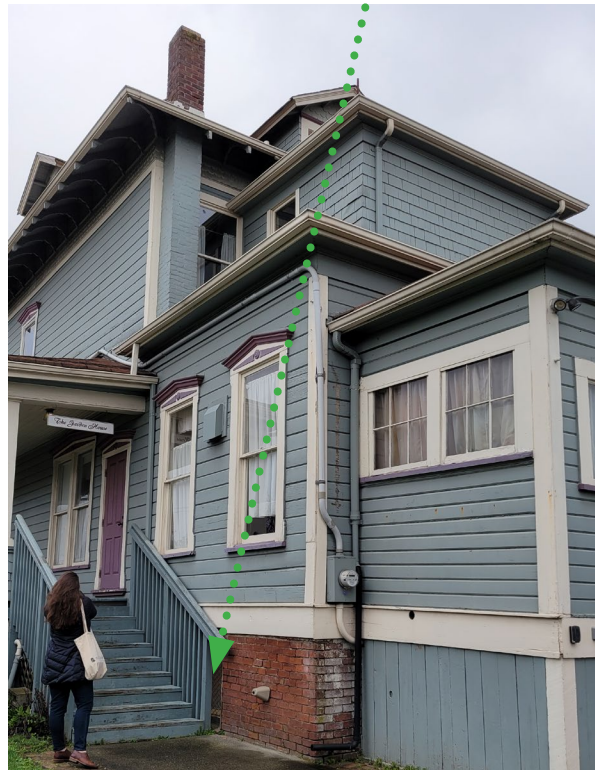
EXISTING BASEMENT WINDOW (#002)
