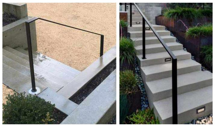
HANDRAIL AT CONCRETE STAIRS COLOR: POWDER COATED BLACK
