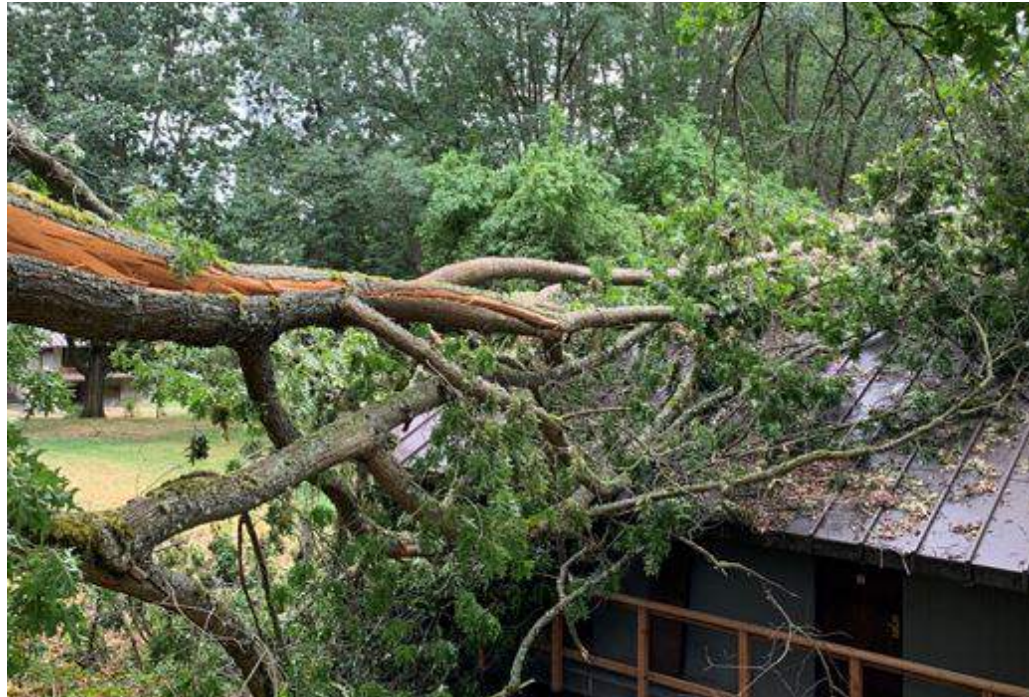
40 trees have failed or died since 2018.
