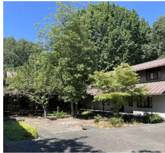
EXISTING CONDITIONS: MIDDLE PLAZA
