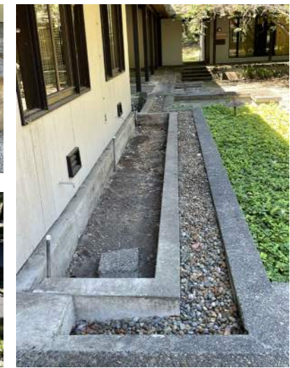
EXISTING CONDITIONS: ROOF DRAIN TROUGH
