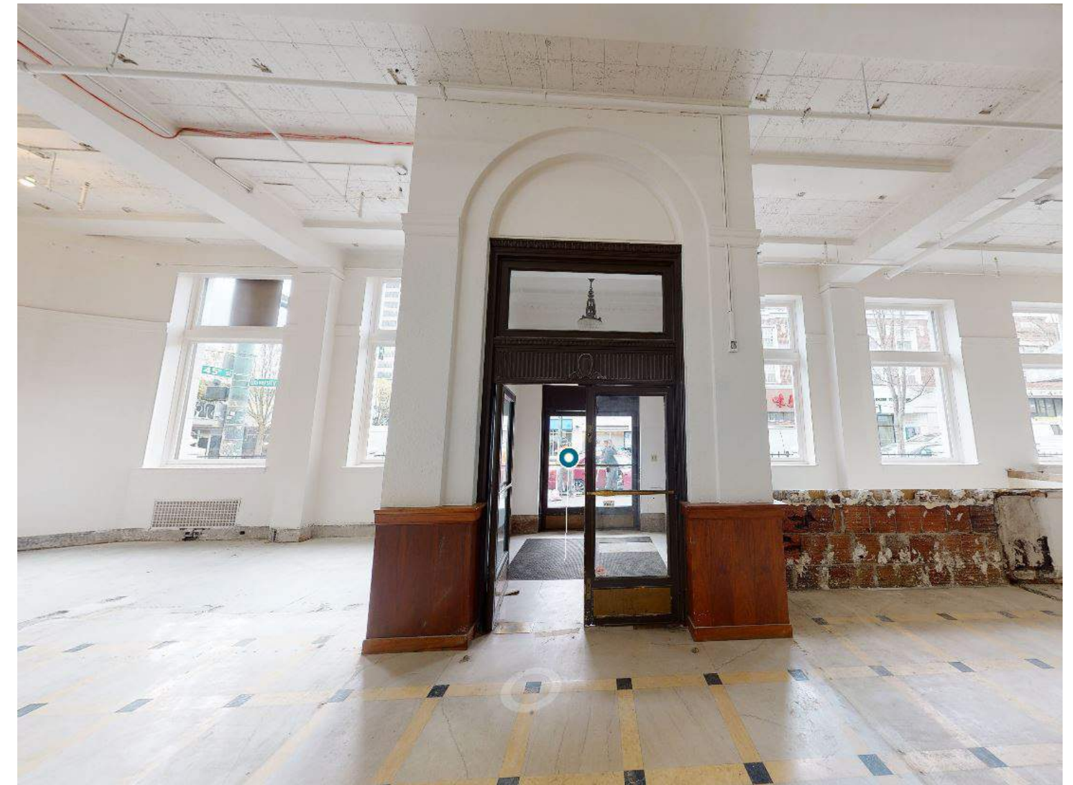
Existing West Vestibule Openings
