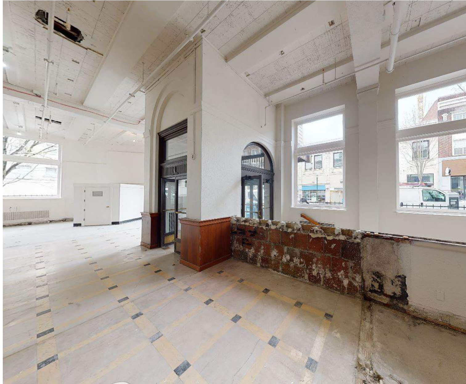
Existing West Vestibule Openings
