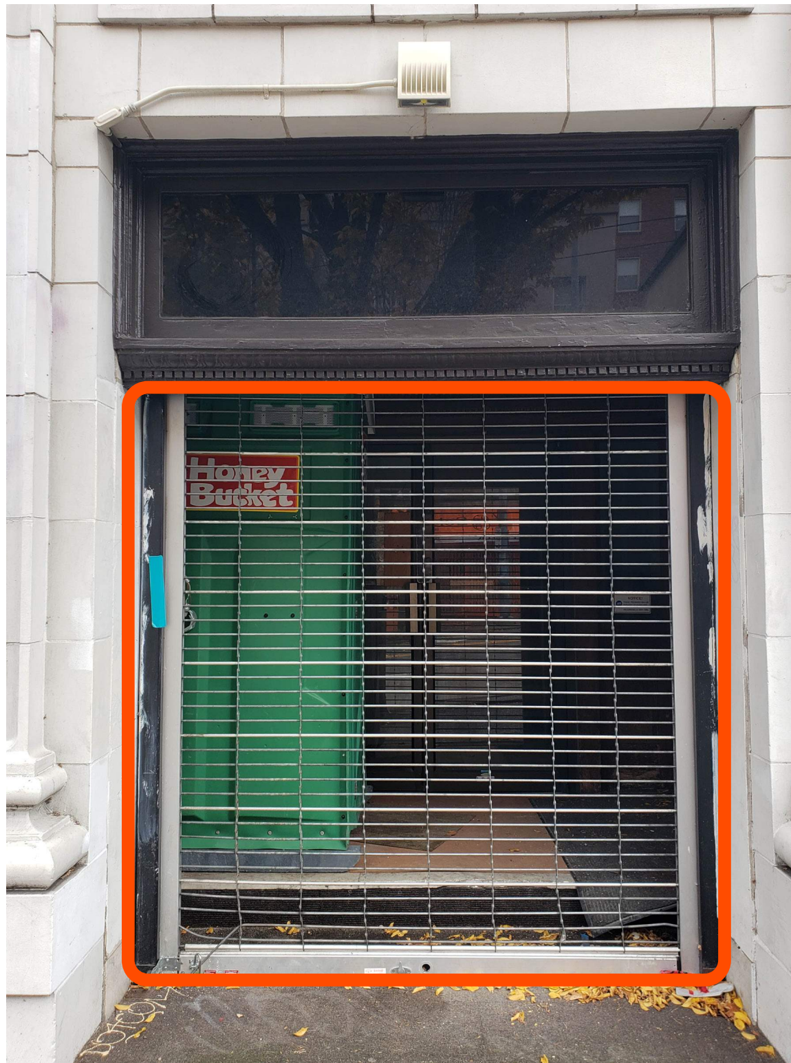
Existing Security Gate at 45th Street Vestibule
