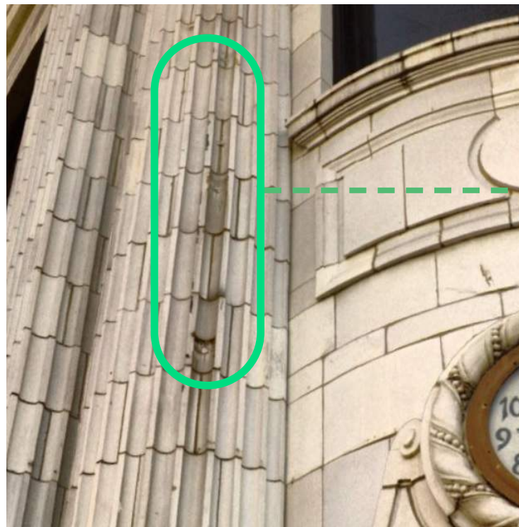
The sign will be mounted within the existing penetrations on the columns from the previous 'Wells Fargo' sign, in order to not add any additional penetrations to the cladding.
