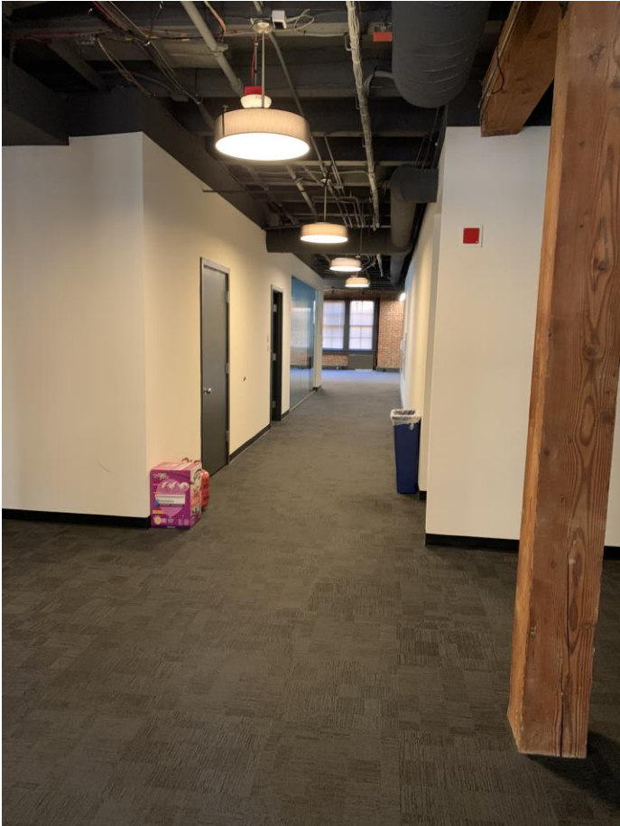
September 2021 – Office Shell
