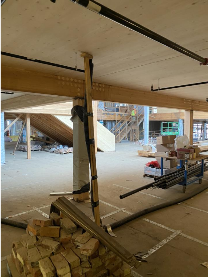
September 2021 – 7 th Floor Demolition
