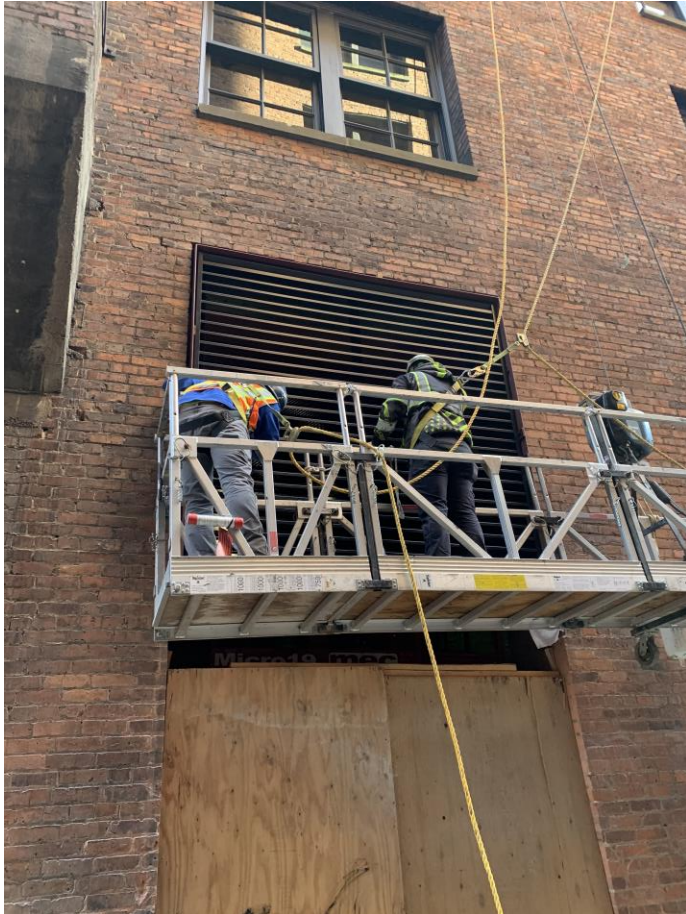
July 2021 – Exterior Work
