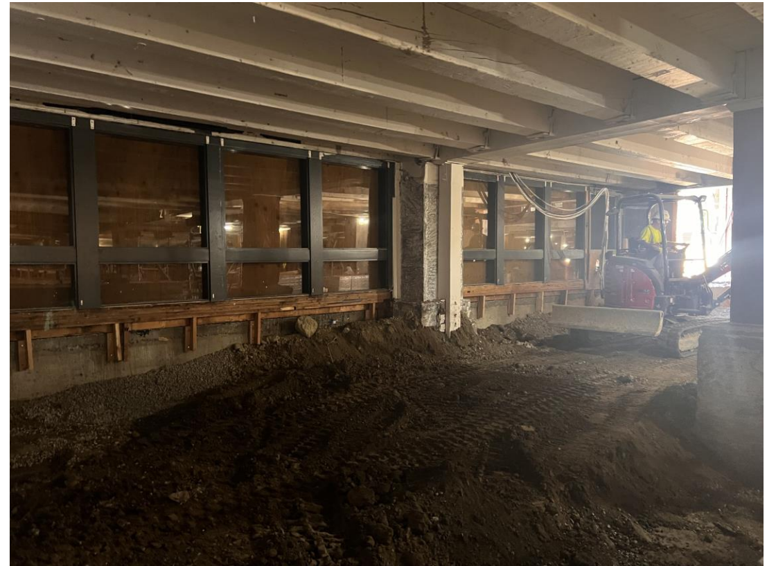
8/2/2023 - Windows and Excavation
