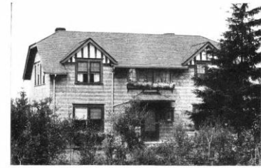
L.—A Shingled House with Alternate Wide and Narrow Coursing of Shingles
