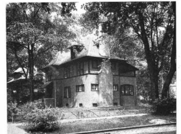
N.—Exterior Plaster to the Ground. No Underpinning shown in this House
