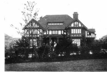
K.—Plaster and Brick
