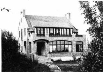
E.—A Pretty Brick House Showing a Tasteful Way to Use Common Brick and Light Mortar
