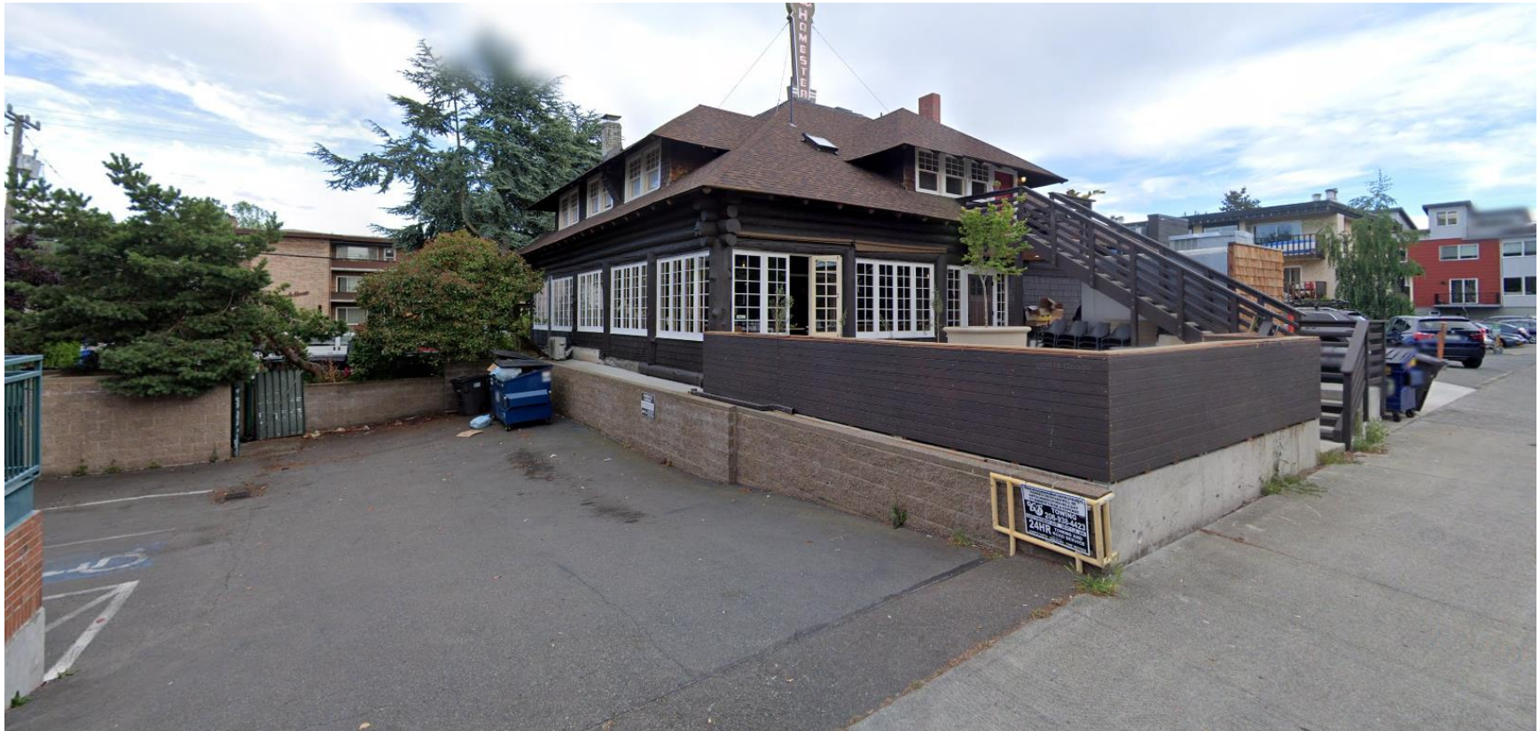
View from alley looking southeast
